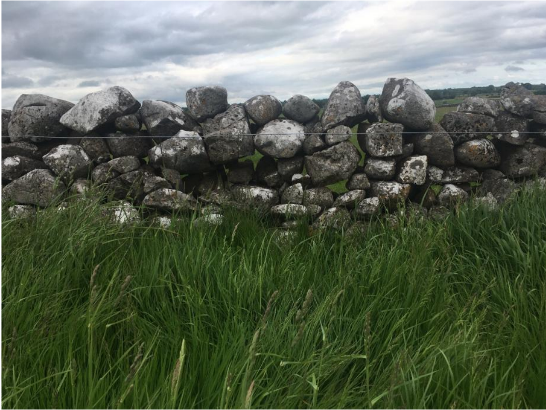
Plate 13-13 East/west oriented wall in the location of Turbine 3, looking north
