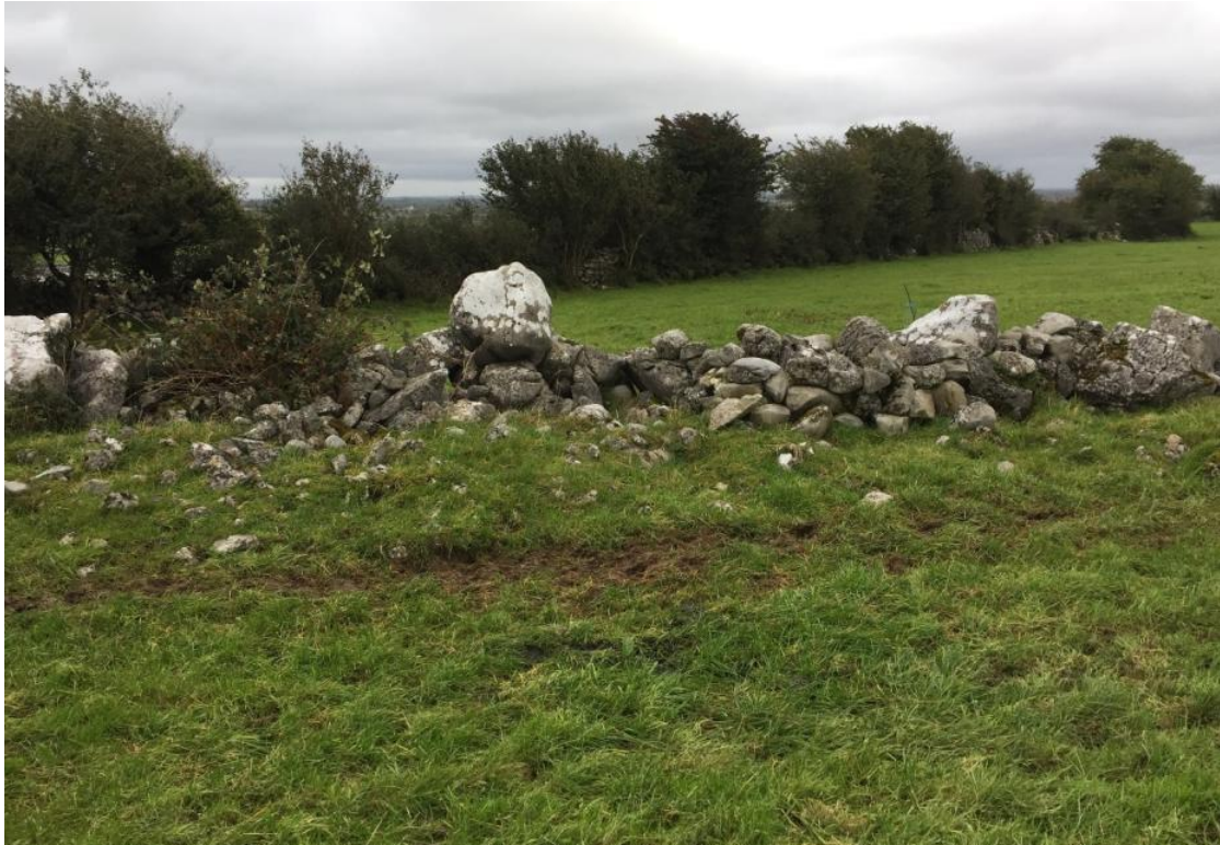
Plate 13-40 North/south oriented wall in the location of Turbine 19, looking east
