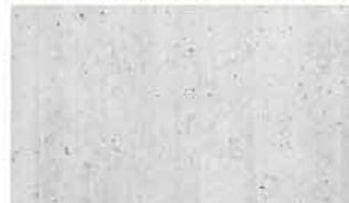
Durable Concrete base
