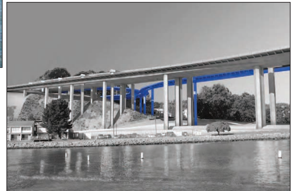
Alternative 2B Ramp Components: Blue highlighting distinguishes Alternative 2B ramp components from SFOBB East Span project components
