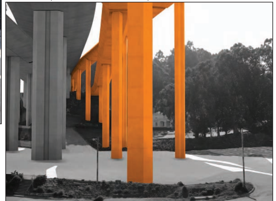
Alternative 4 Ramp Components: Orange highlighting distinguishes Alternative 4 ramp components from SFOBB East Span project components
