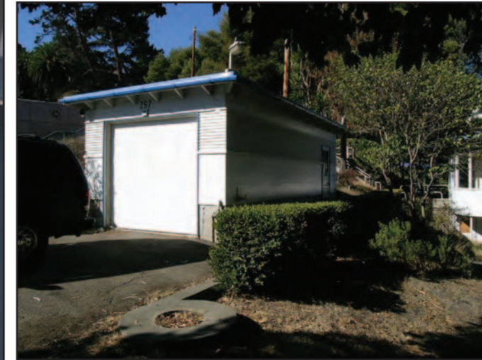
Building 267 to be removed as part of Alt. 2B
