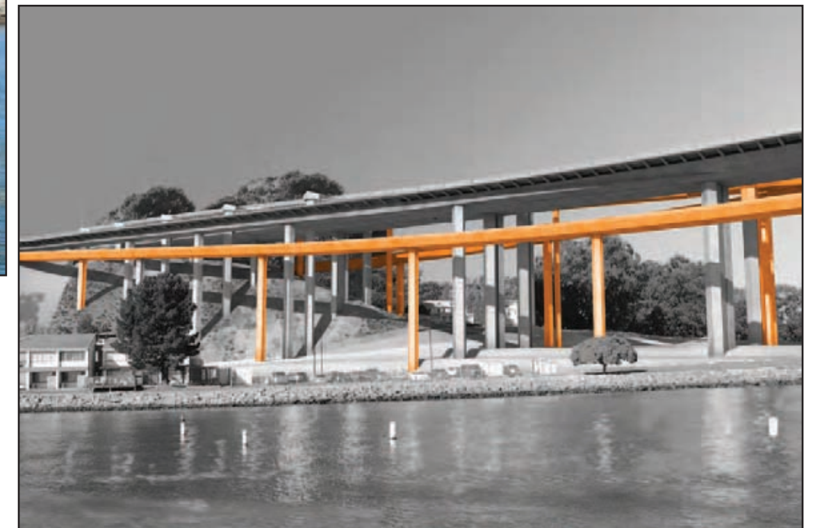
Alternative 4 Ramp Components: Orange highlighting distinguishes Alternative 4 ramp components from SFOBB East Span project components
