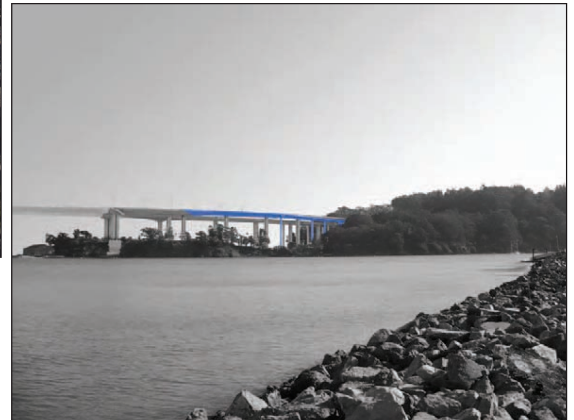
Alternative 2B Ramp Components: Blue highlighting distinguishes Alternative 2B ramp components from SFOBB East Span project components
