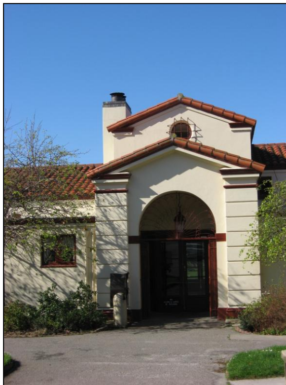
Photograph 7: East entrance to clubhouse, camera facing west, 3/4/2010
