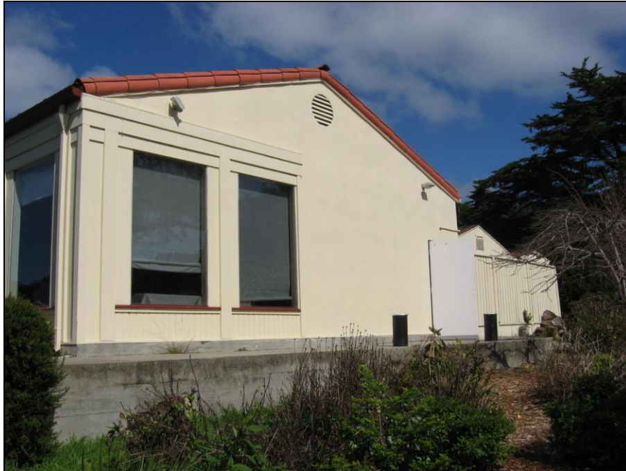
Photograph 8: South side of clubhouse, camera facing northeast 3/4/2010
