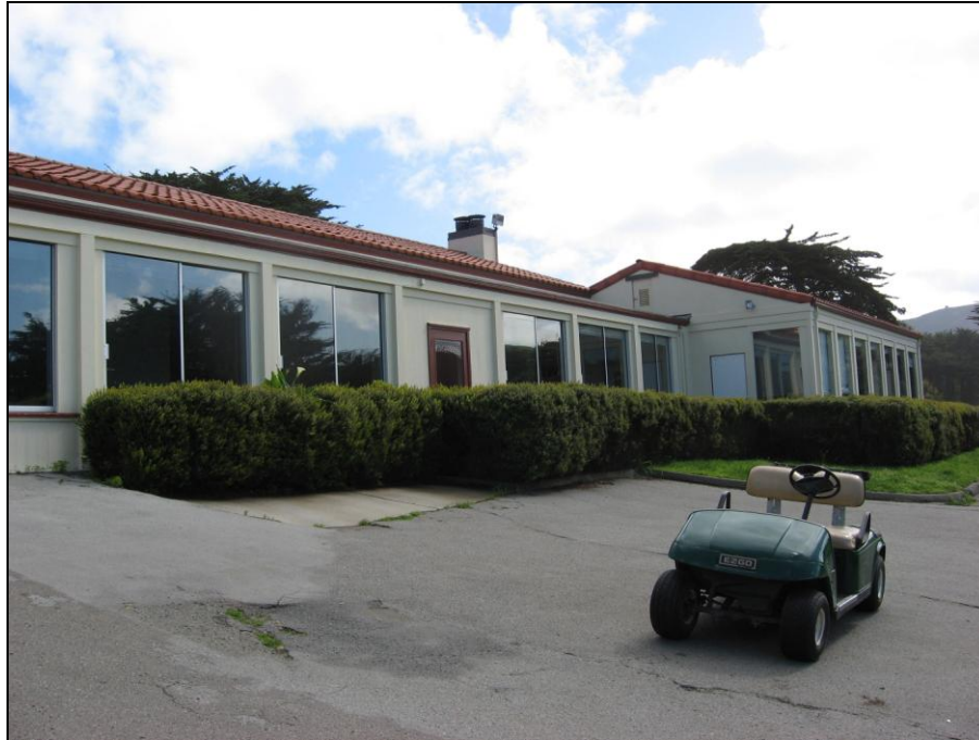
Photograph 10: West side of clubhouse, camera facing southeast 3/4/2010
