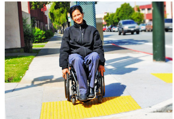
Truncated domes at edge of vehicular zone
