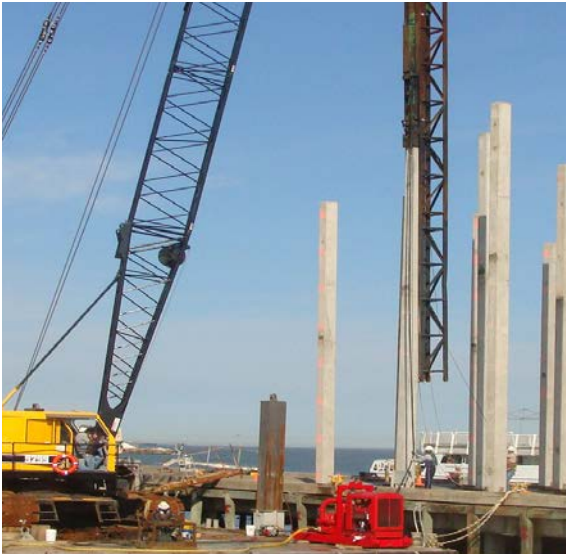
Pile driving during appropriate times of the year.
