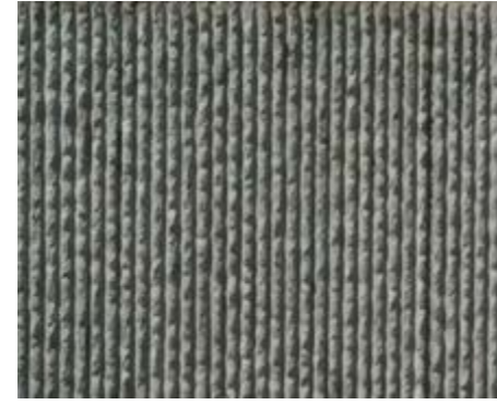
Concrete - form finished
