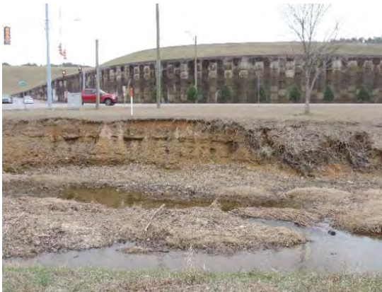
Figure 5.2: Streambank Erosion in Irondale, Shades Creek Watershed
