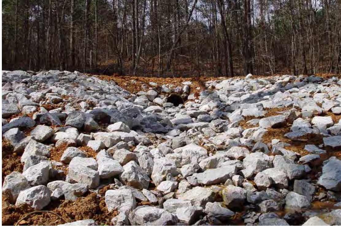
Proper culvert installation.
