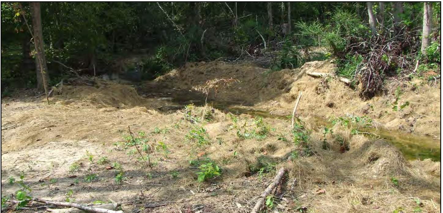
Cleared stream crossing, stabilized with hay.
