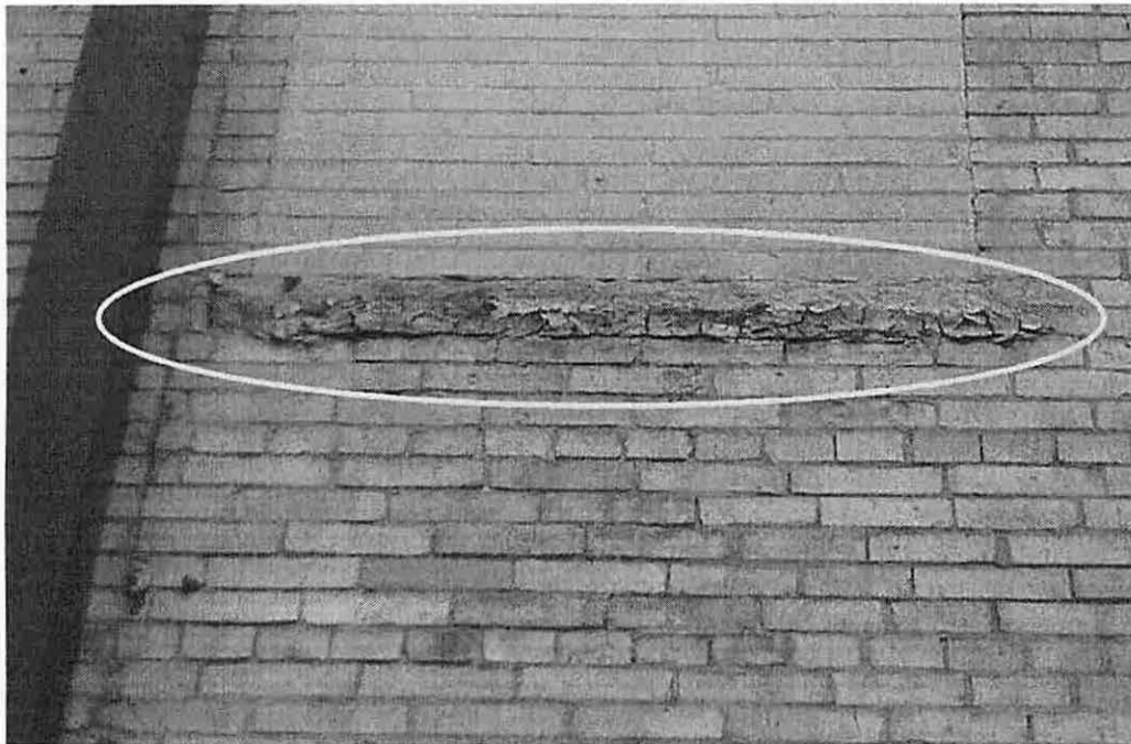
Figure 35: Deteriorated sill.
