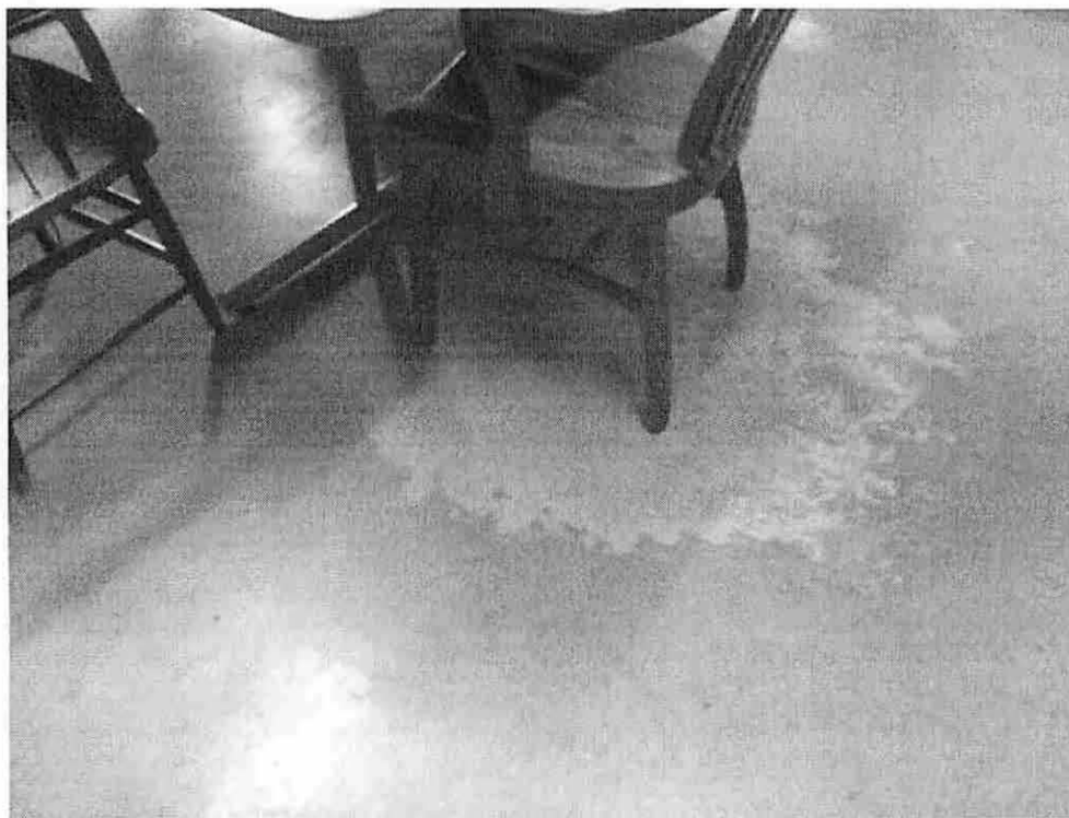
Figure 48: First floor concrete flooring.
