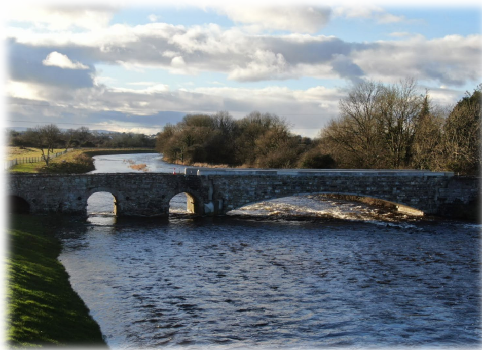
Dunkellin River & Aggard Stream Flood Relief Scheme – Completed Works at Dunkellin bridge
