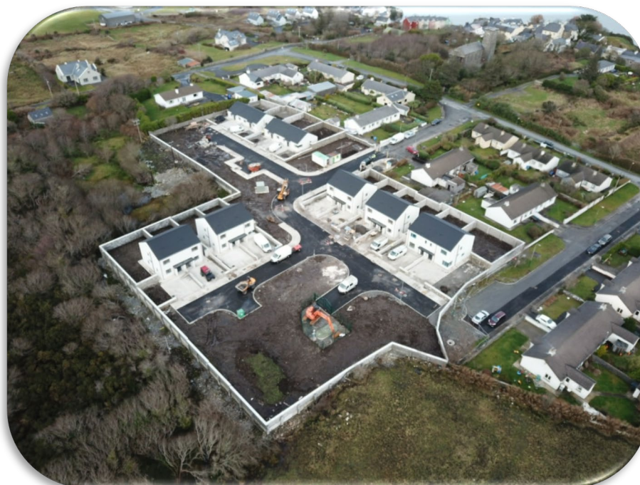
Cnoc na Carraige, Roundstone – under construction
