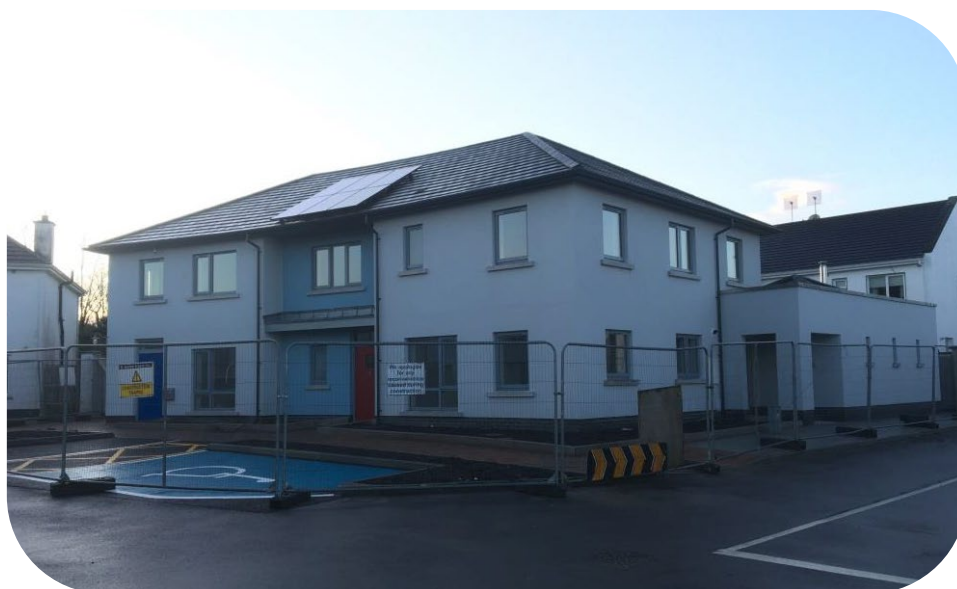
Finishing Disability Access Units – Esker Fields, Ballinasloe
