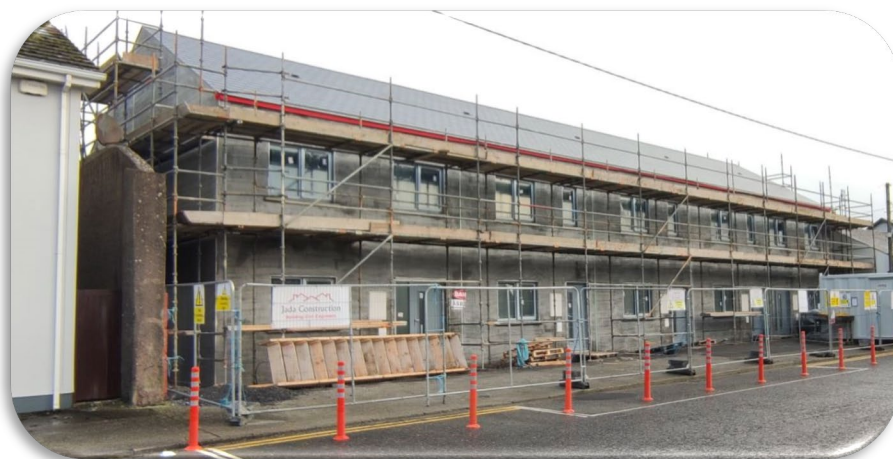
Plás an Iarla, Barrack Street, Loughrea – under construction
