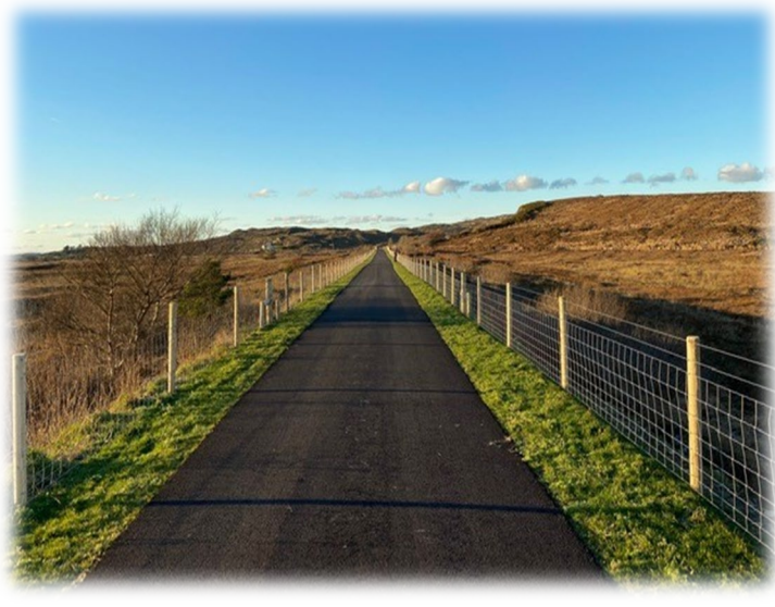
Connemara Greenway at Derryvickrune & Gowlan
