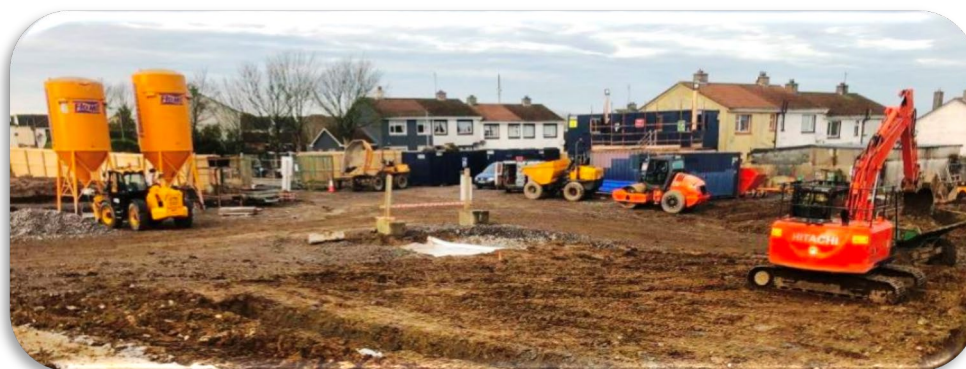
Fána Bhuí, Tuam – under construction
