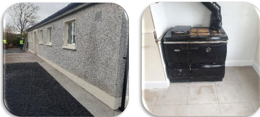
Major renovation works completed at traveller specific accommodation at Canal Drive, Ballinasloe
