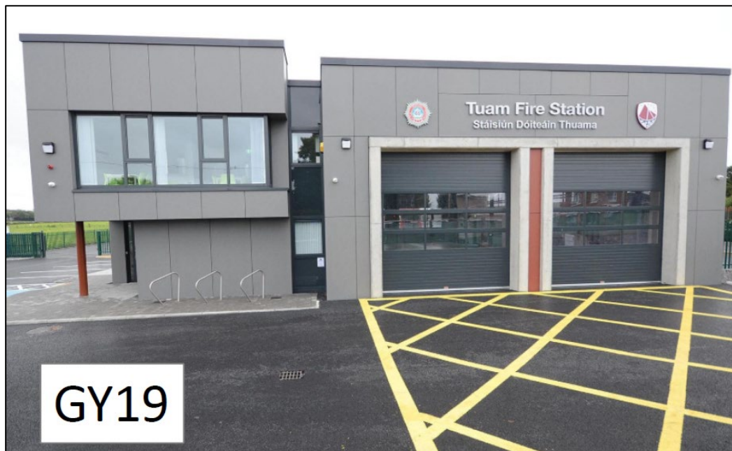
Figure 2: New Fire Station in Tuam Operational October 2018
