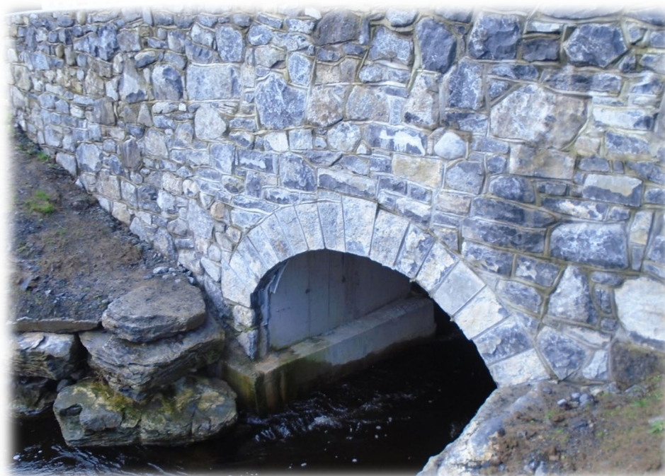
Cloondahamper Bridge, Tuam completed in 2020
