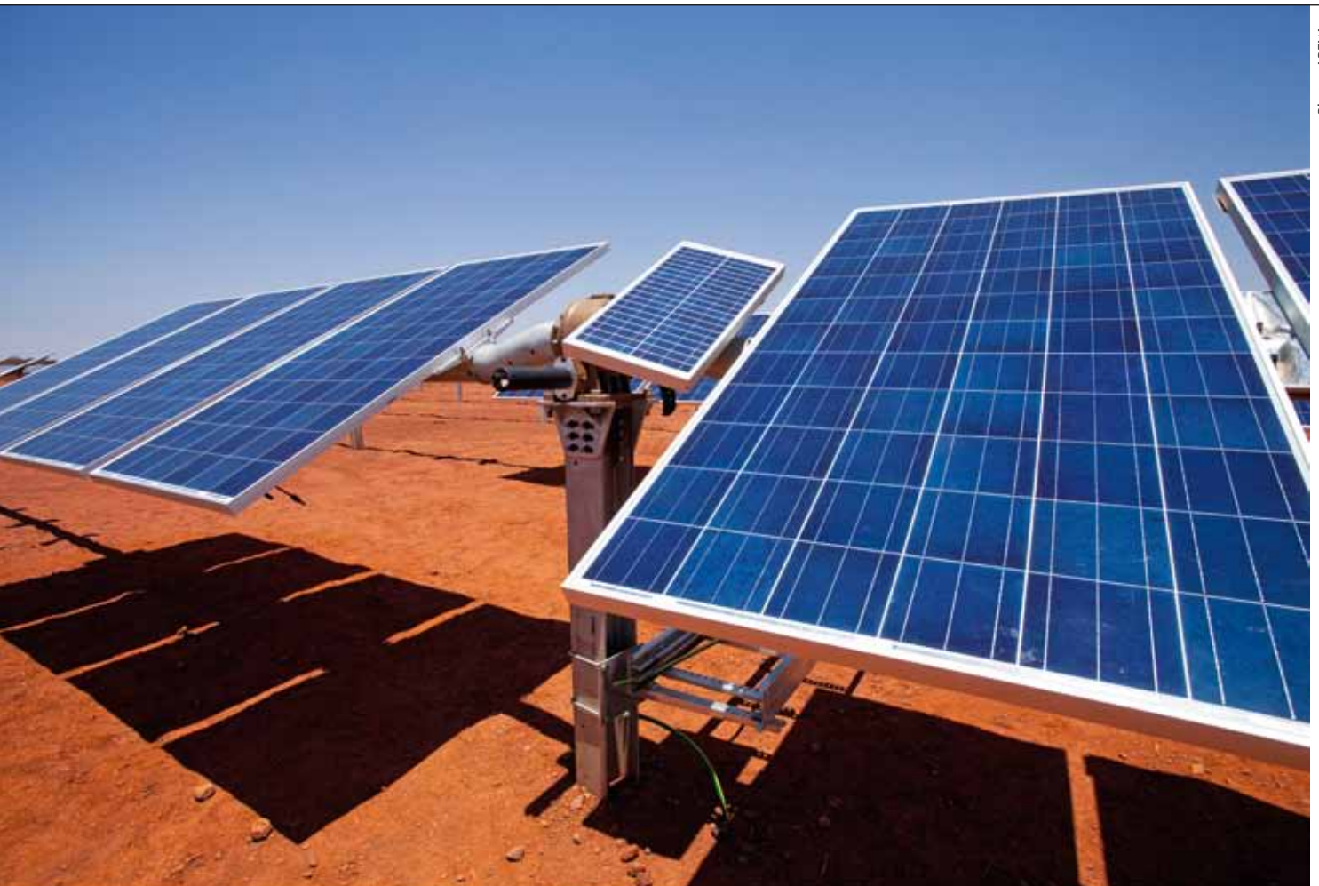
U.S. tracking provider Nextracker supplied the self-powered dual axis system at the DeGrussa mine. The trackers will have to tolerate extreme temperatures and dry and dusty conditions.
