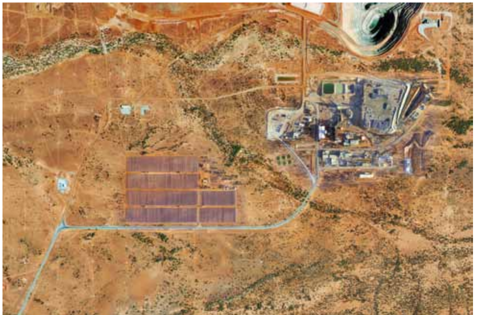
Located adjacent to the open cut and underground mine, the solar+storage array will be able to supply the operation completely with power during daylight hours.
