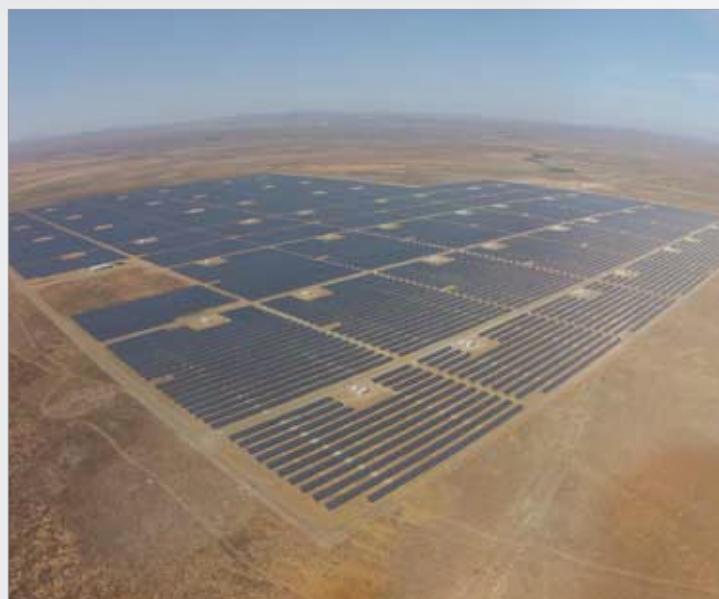
Sterling and Wilson was the EPC for this 90 MW solar PV plant located in South Africa.
