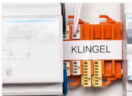
DIN-35 rail-mount application (residential door bell)
