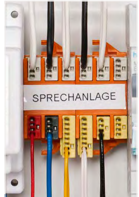
Example of a residential intercom application
