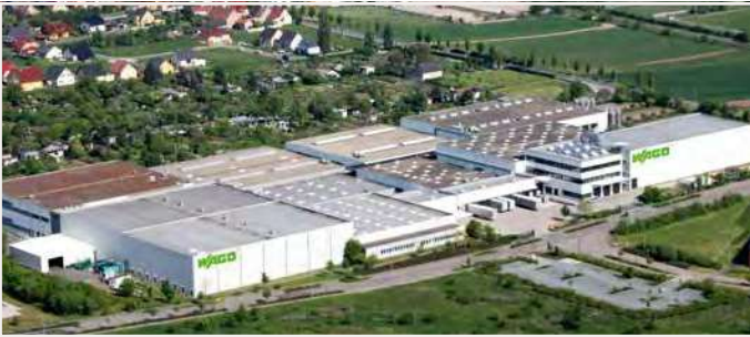
WAGO Sondershausen, Germany
