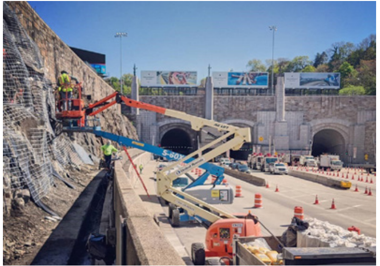
Rock slope stabilization in New Jersey at the Lincoln Tunnel.
