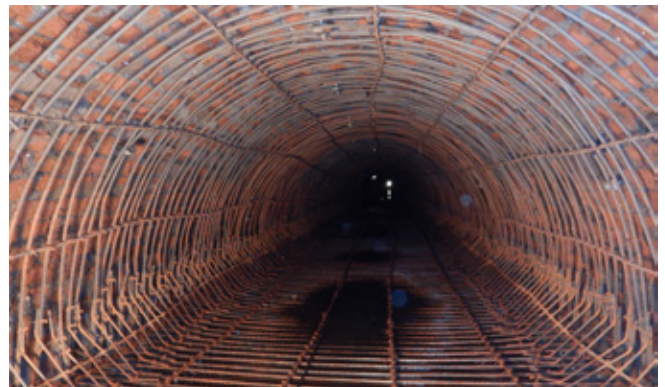
Fig. 8: Fixing steel reinforcement
