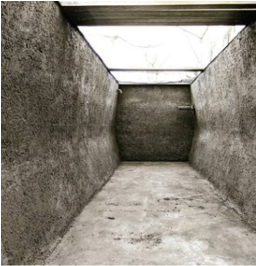
Wet-mix shotcrete lining for tank of an on-site wastewater treatment plant, 10" thick - It's all about perspective.
