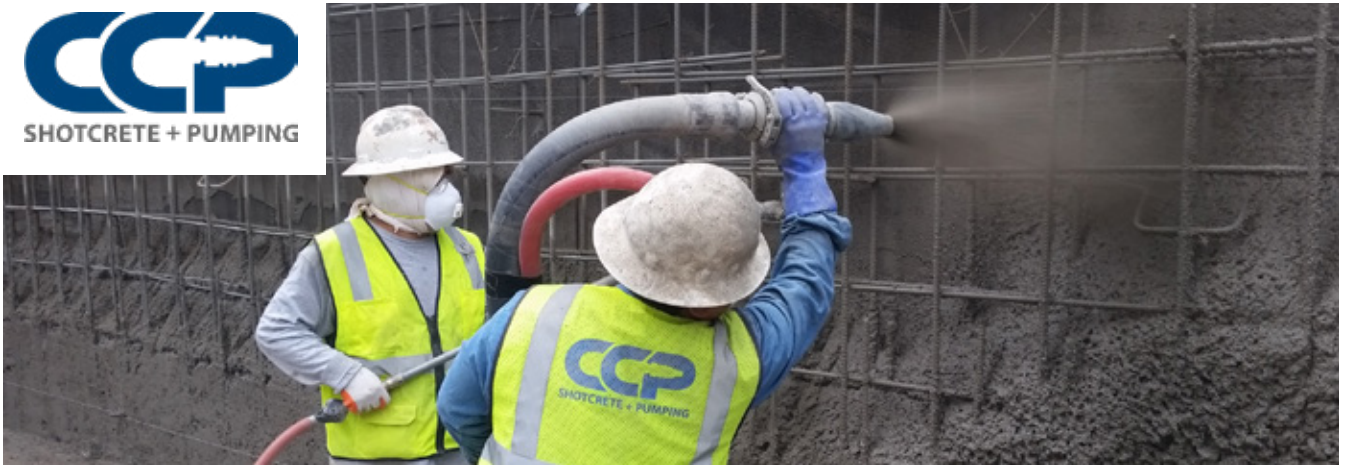
Fig. 1: Shotcrete basement walls in high density urban environments – Dallas-Fort Worth.
