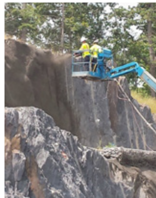
Newburgh Water Tunnel Bypass Project; a rock stabilization job. The production line for 5000 PSI wet-mix ran up to 60' above the ground, holding back the earth for the new access road for an aqueduct tunnel providing potable water to the residents of New York City.
