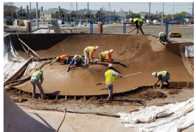
Fig. 4: Steel trowel finish shotcrete skate park bowl
