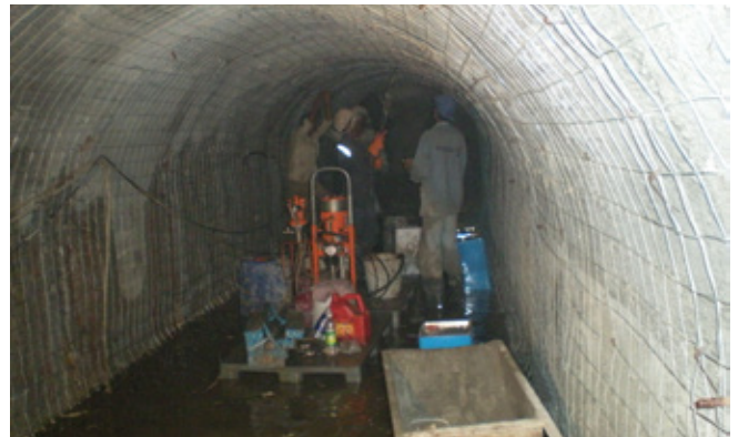
Fig. 7: Installed ports for injecting 2-component rigid polyurethane resin
