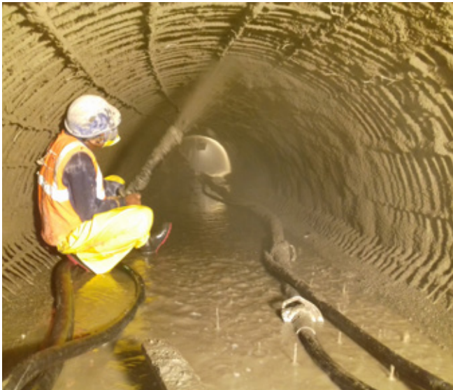
Fig. 9: Placing wet-mix shotcrete
