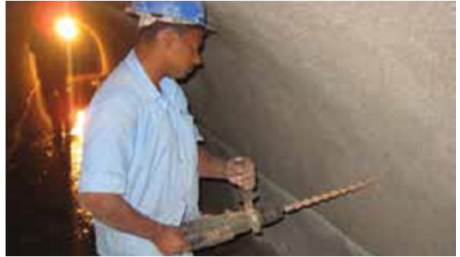
Fig. 10: Drilling holes into the brick masonry
