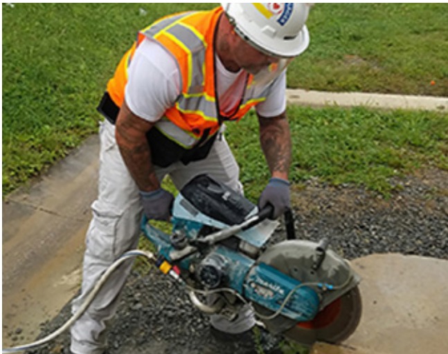
Figure 1: Using water with a cutoff saw when cutting materials that contain crystalline silica substantially reduces the amount of dust created during these operations.
