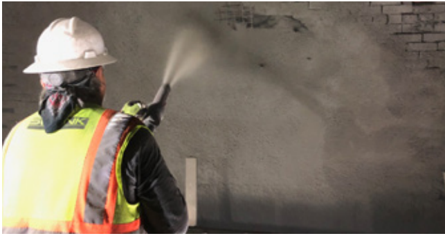
Railroad Tunnel Shotcrete Repair
