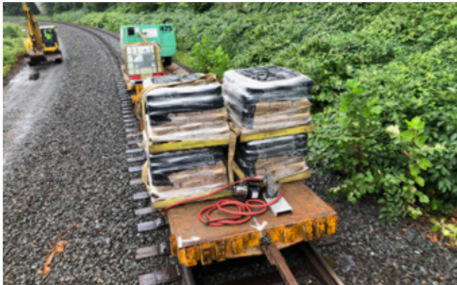
Emergency Tunnel Repairs
