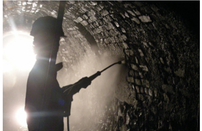
Fig. 6: High-pressure waterjet washing
