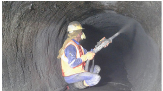
Fig. 12: Spraying two-component mineral-based mortar system to form a lining
