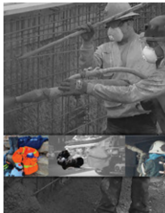
On the cover: Main photo, Shotcreting a curved retaining wall.
