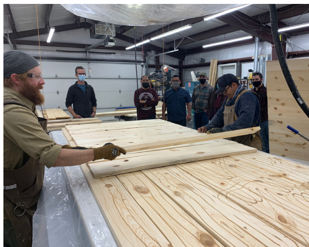
Manual layup of a CLT panel (Photo courtesy of TimberAge)
