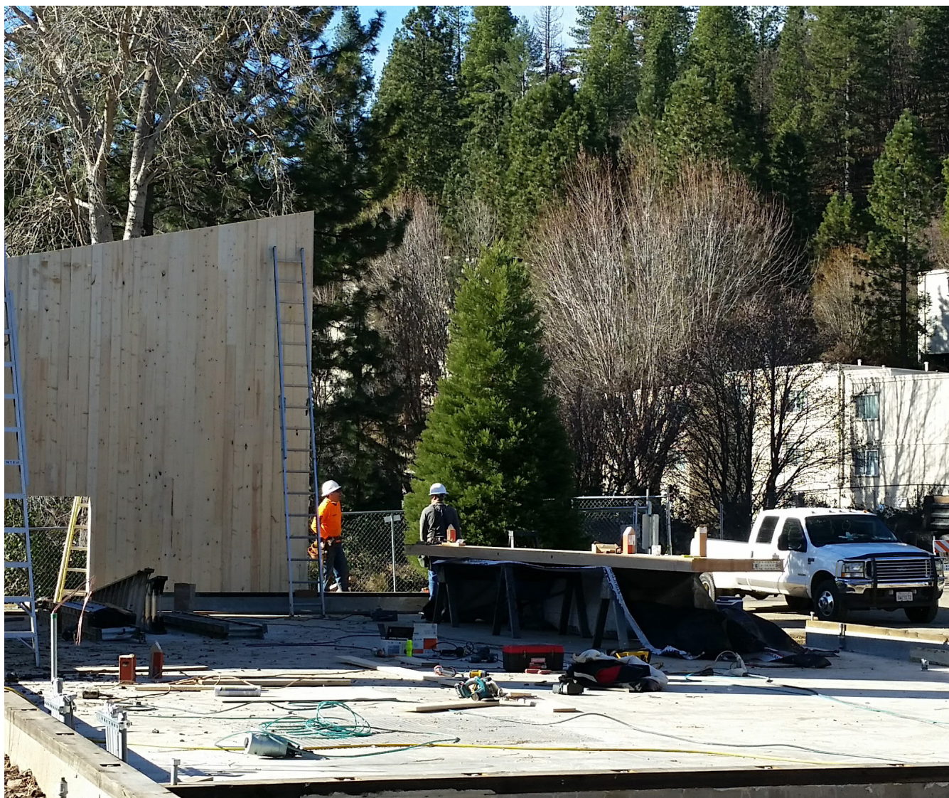
First cross laminated timber building in the State of California, under construction, Quincy, CA.
