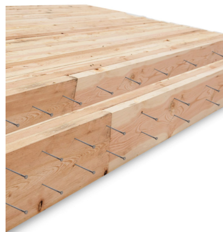
Figure 4. Nail-laminated timber. Image courtesy of ThinkWood ( https://www.thinkwood.com/mass-timber/nlt )
