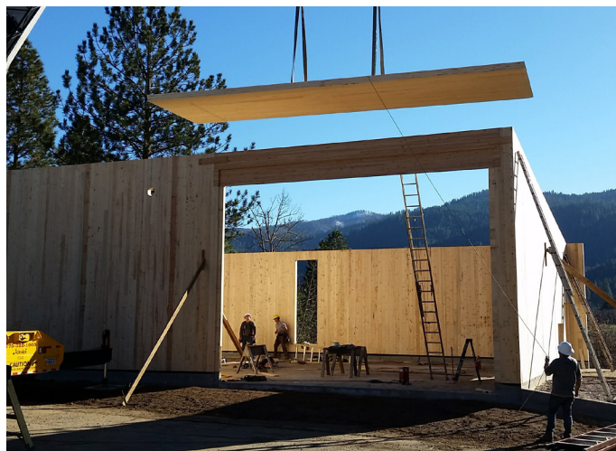
CLT building in construction in Quincy
