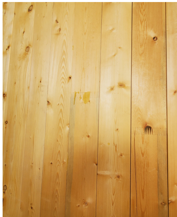
A CLT wall with finger joints
