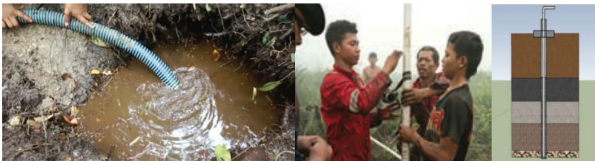
Figure 70. Drilling well construction process.
