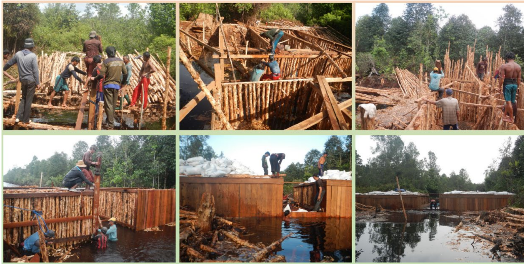
Figure 64. Canal-blocking construction process in Sebangau National Park.
