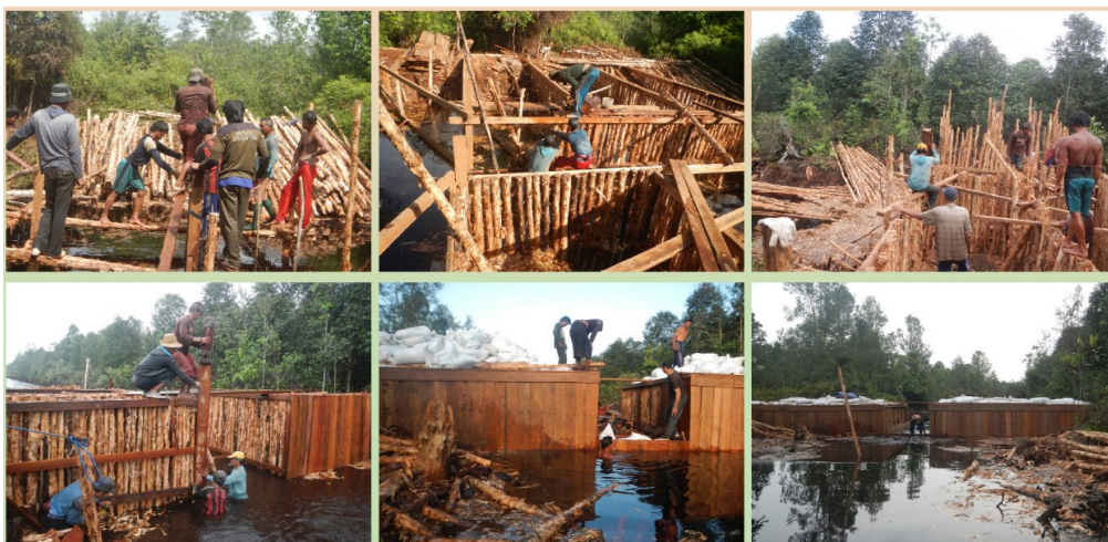
Figure 79. Canal-blocking construction process in Sebangau National Park.
