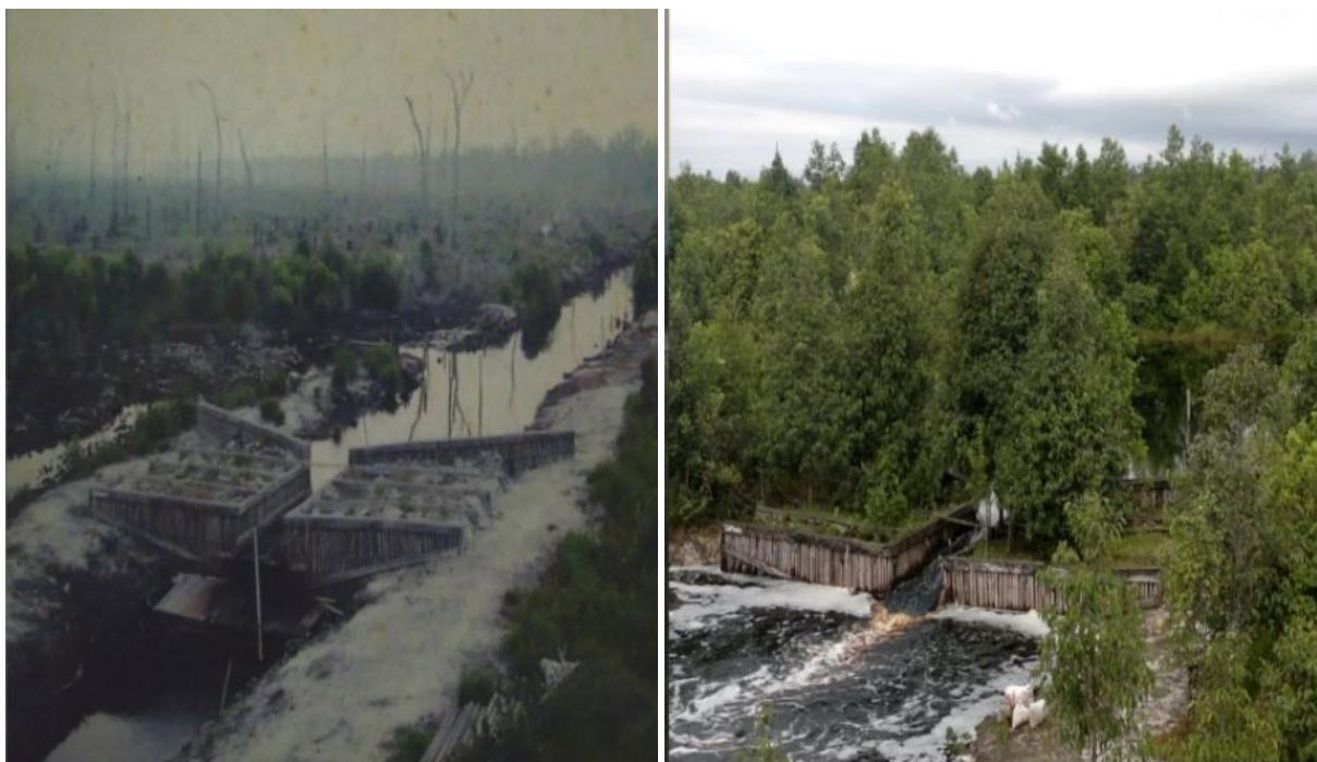
Figure 83. Photo of the success of canal blocking construction in Sebangau National Park
