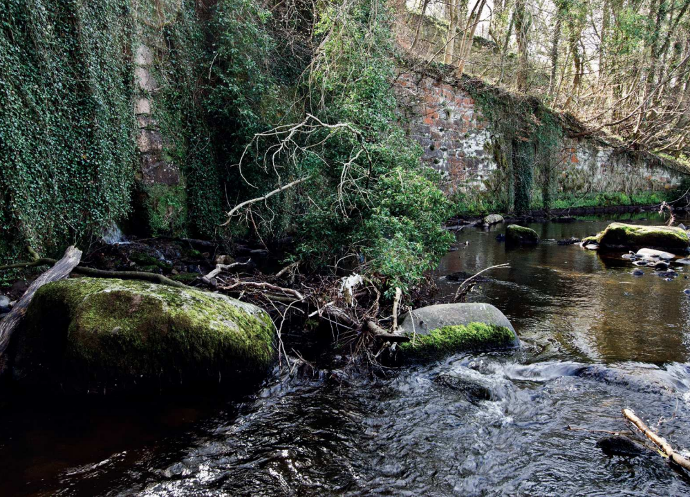
Lower Bowling Green Wall – Girdle Traverse
