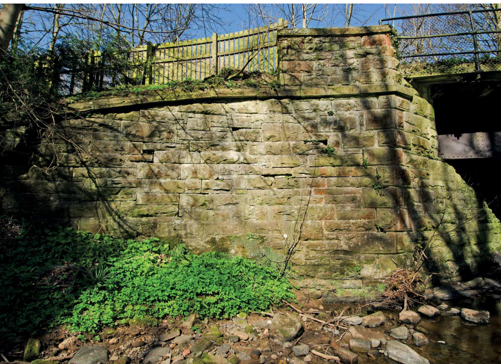
Tannery Bridge – Spike Wall
