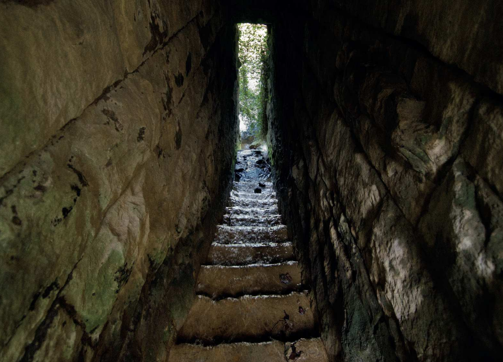
Lower Bowling Green Wall – 'descend wet stairs'
