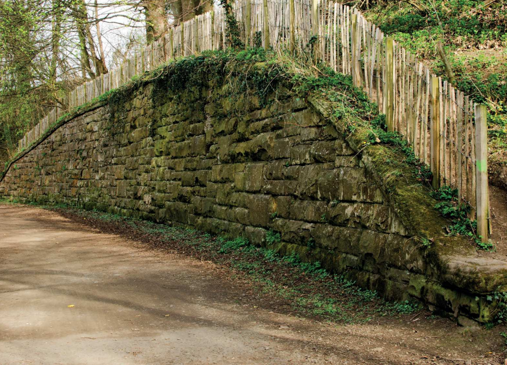
Upper Bowling Green Wall
