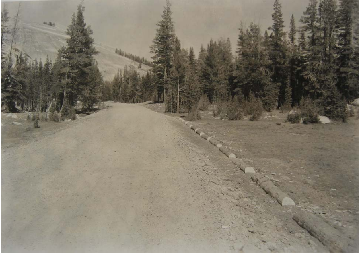
Figure 1-4. The realigned Tioga Pass Road through Tuolumne Meadows, under construction in 1935. Note small lodgepole pines near the road, but not significant numbers of seedlings in bare areas along the shoulder. Negative number ECW1311. Source: Yosemite Research Library.
