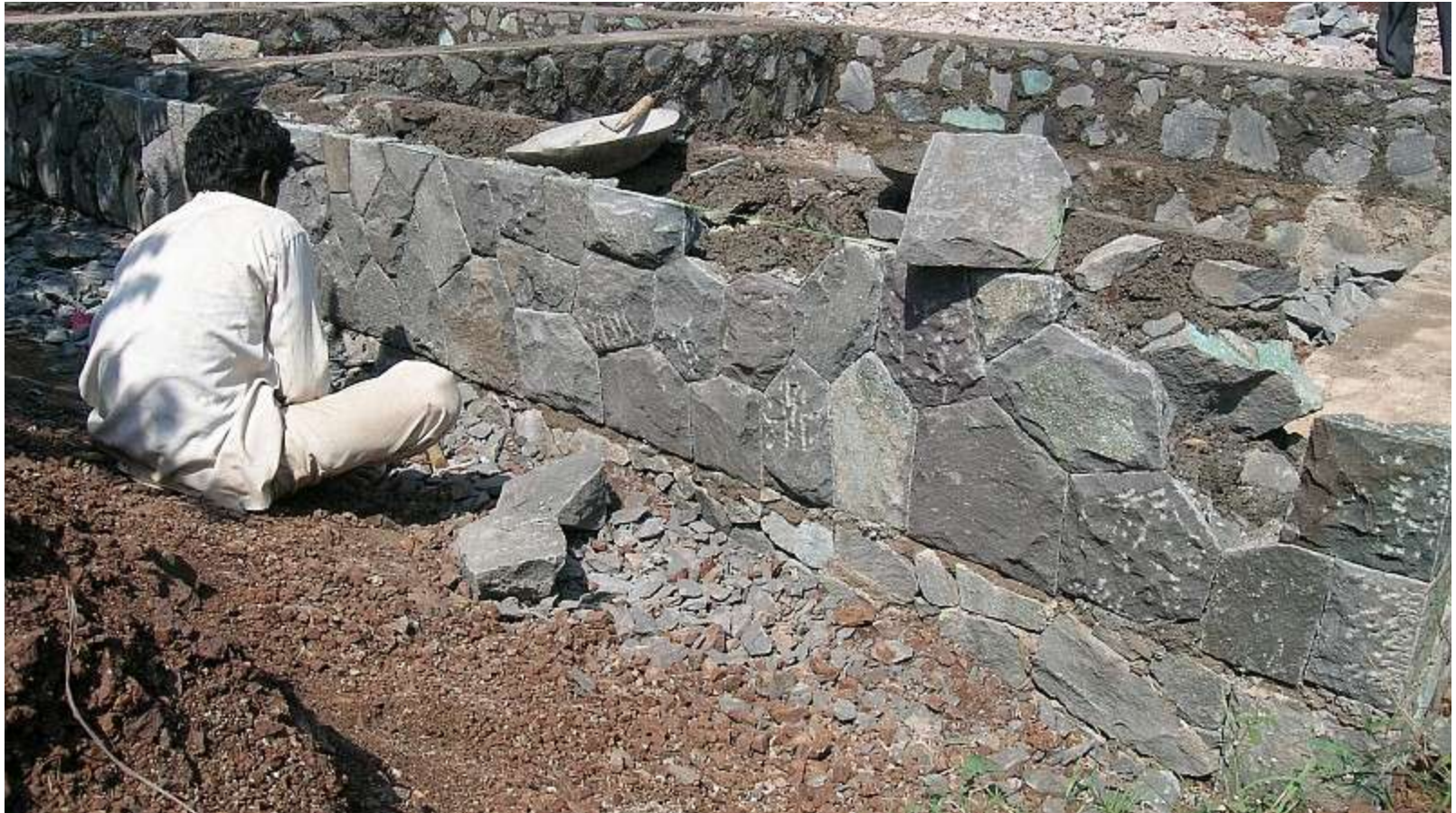
Plinth in Random Rubble Masonry to receive A Load-Bearing wall Above.
