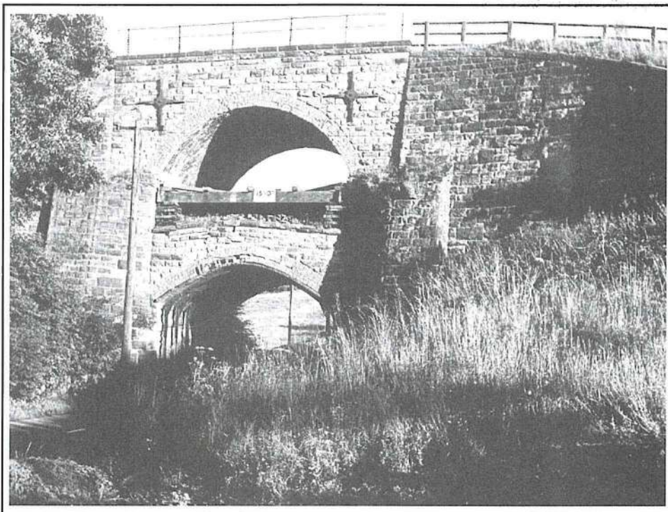
The Claphow double-arched bridge on Stanghow Road - now demolished
