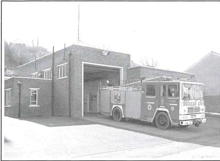
Skelton Fire Station
