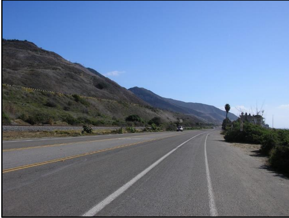
Figure 3.1-3. View along PCH from the Project Site Looking East
