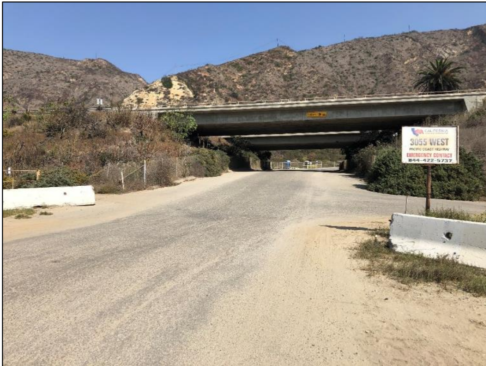
Figure 3.4-8. Onshore Pipeline Segment Developed Lands Looking North
