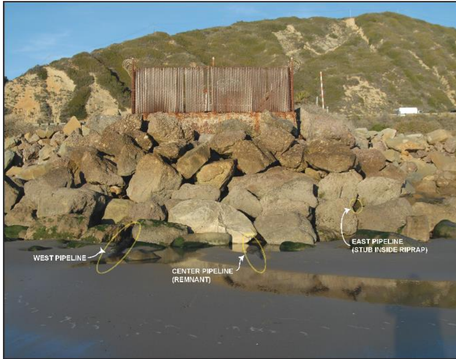
Figure 2-2. Onshore Project Components at Low Tide (South Elevation)
