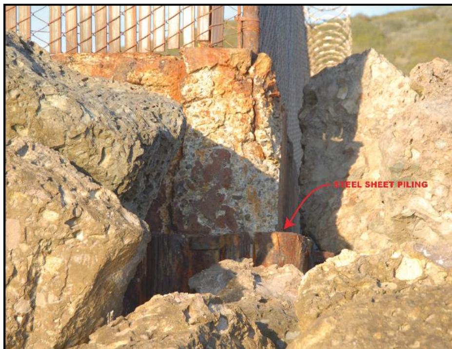
Figure 2-3. Steel Sheet Piling Foundation at Concrete Vault
