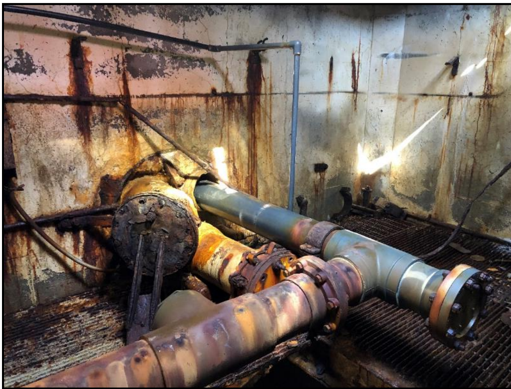
Figure 2-6. View of the 36-Inch Casing Inside the Vault Enclosure
