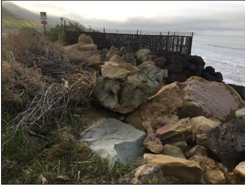
Figure 3.4-7. Rip Rap and Ruderal Habitat Adjacent to Vault Structure Looking East
