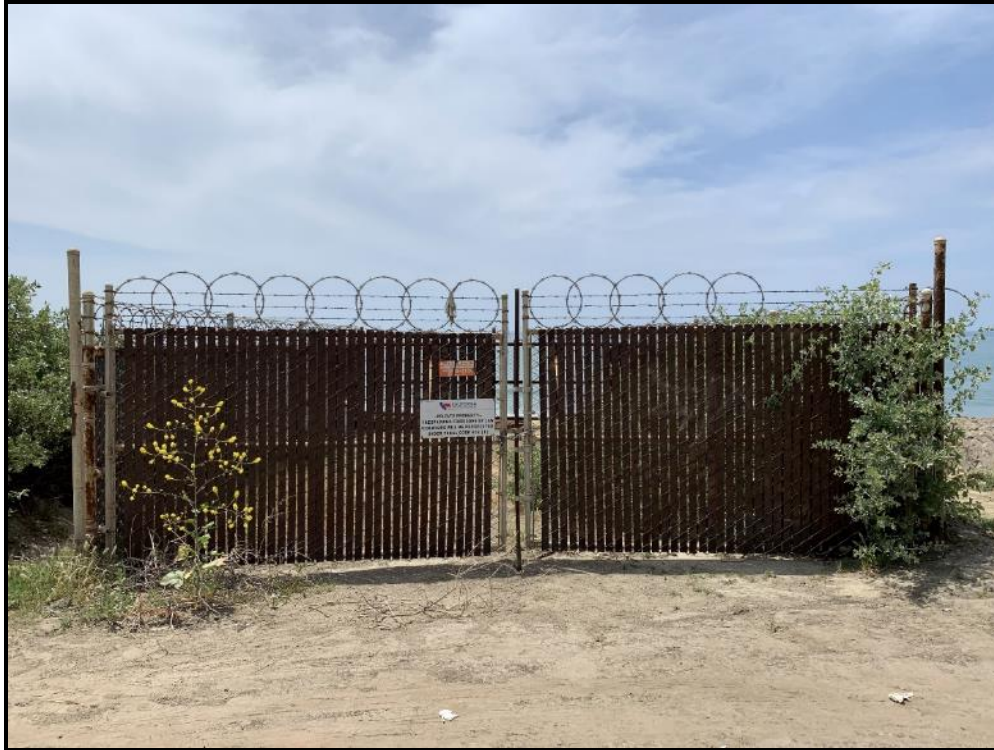
Figure 2-4. View of Vault Entrance and Staging Area Looking Southwest
