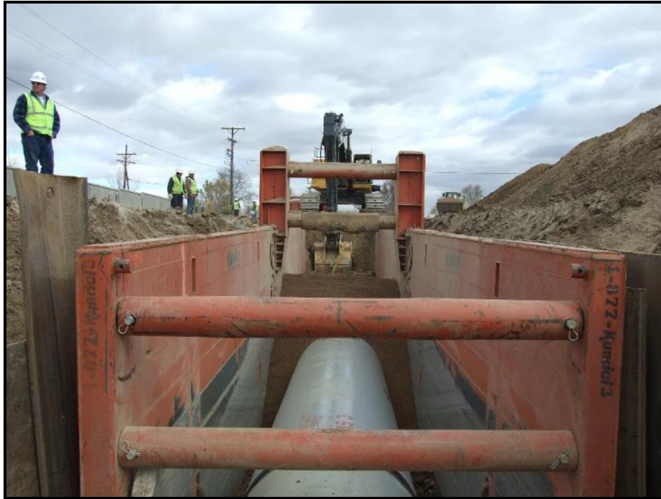
Figure 2-12. Example Trench Box Installed
