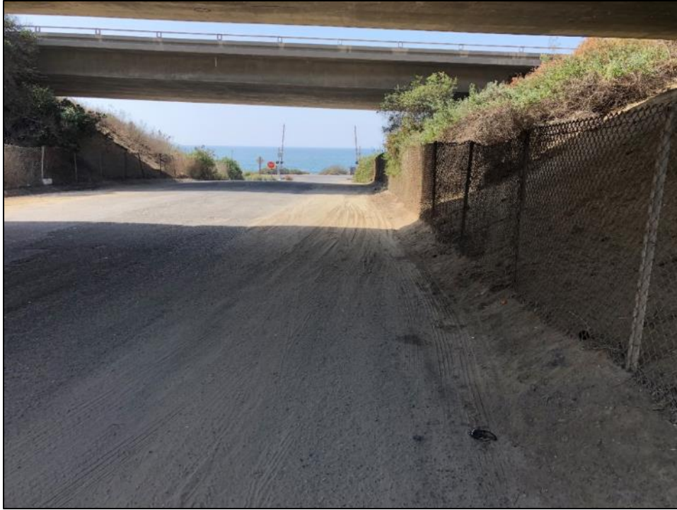
Figure 3.4-9. Onshore Pipeline Segment Developed Lands Looking South
