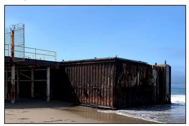
Figure 2-3. 421-1 Sheet Pile Conditions (West and Northern Walls)
