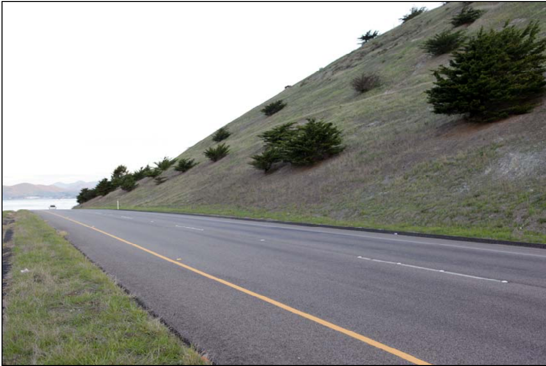
Figure F-A.2a. KVA 4 – Existing View
