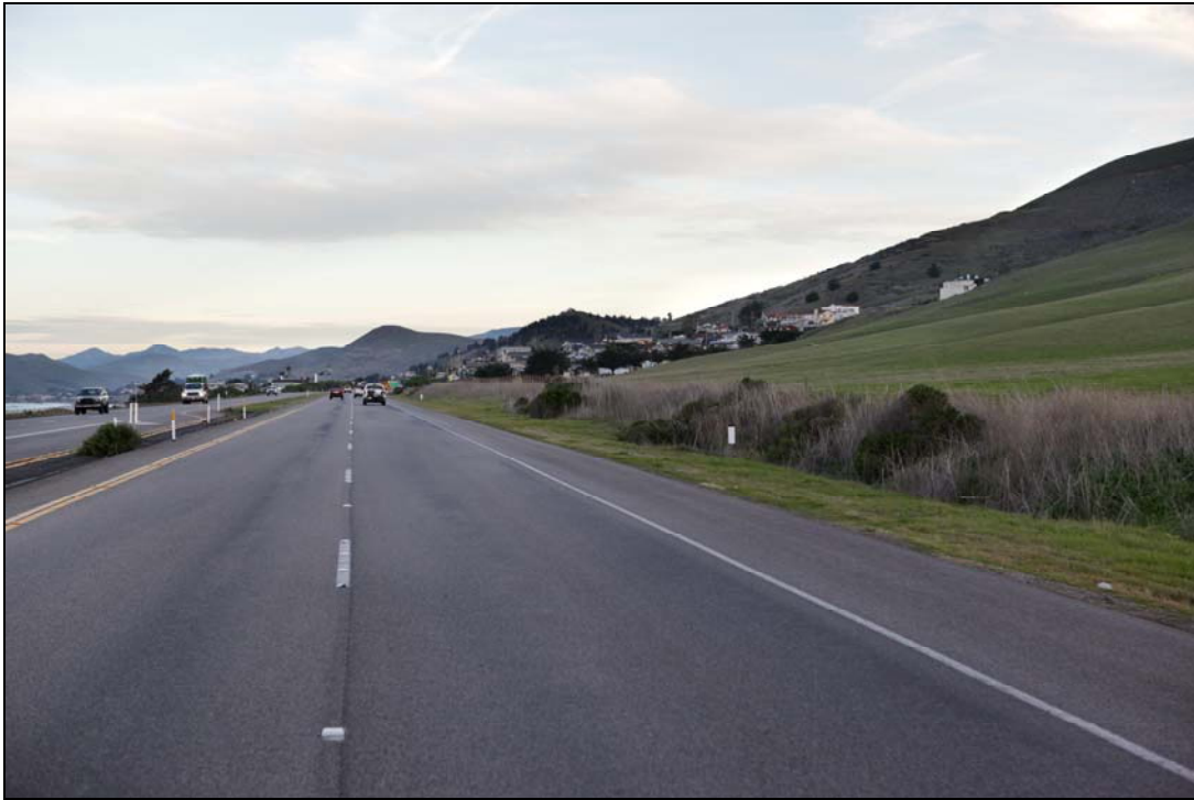
Figure F-A.3a. KVA 5 – Existing View
