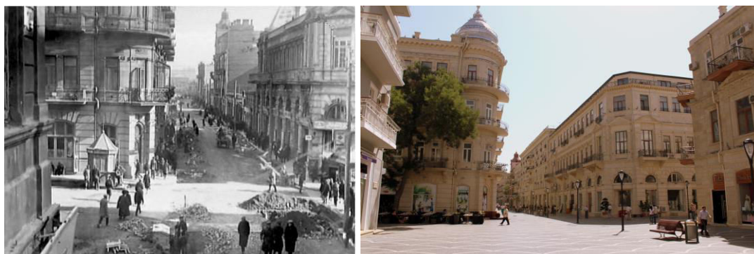
Pic.1 Nizami Street (Baku, Azerbaijan)
