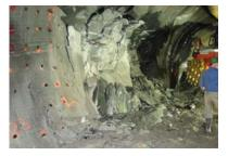
concrete and reinforced concrete. Dā-mite is mixed with water and placed in predrilled holes, where it sets and expands with a compressive strength of over 18,000 PSI, Dā-mite has more than enough force to get the job done. No license or permits are required. There are four grades of Dā-mite, providing enough versatility to be utilized in drilled hole diameters from 1" to 2 3/4". www.da-maite.com
