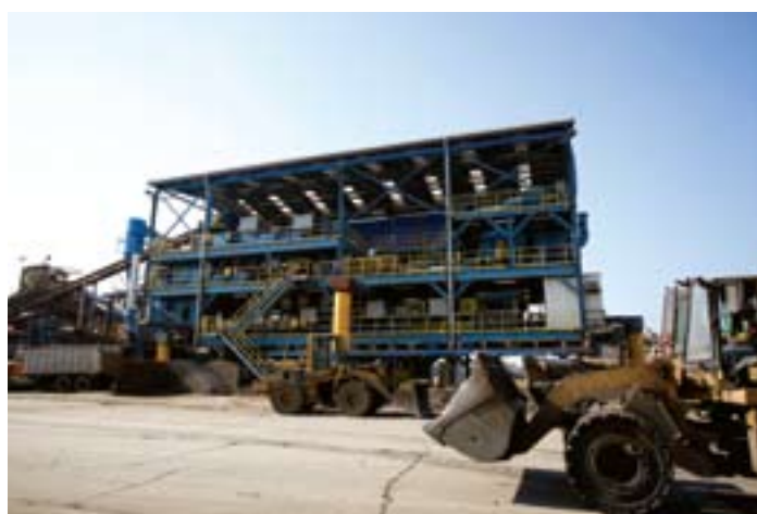
New state-of-the-art non-ferrous shredder residue plant at Claremont Terminal, Jersey City, NJ, USA.
