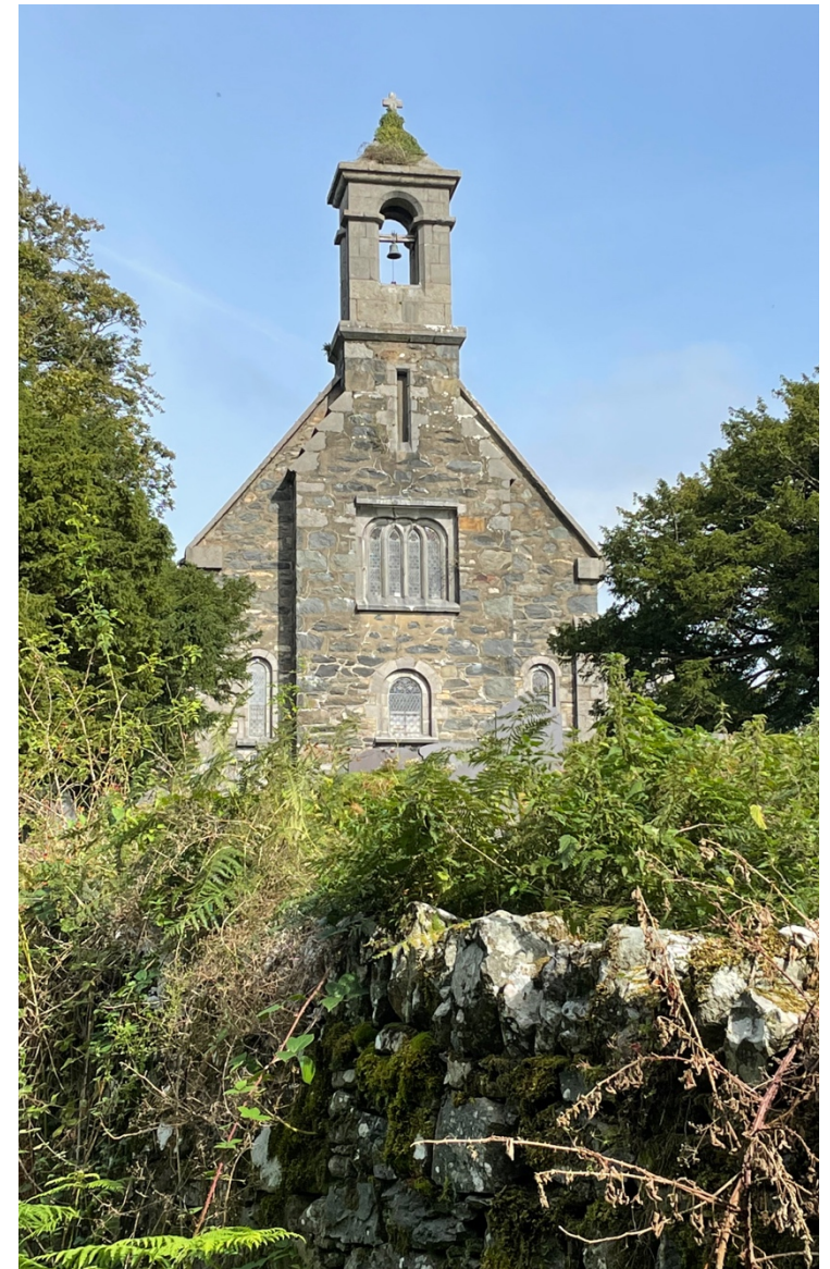
01 View of St. Llechid's Church from beside Afon y Llan
