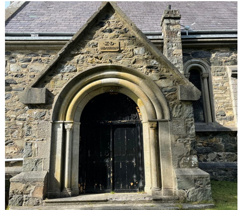
31 St Llechid's Church, Potential for a new community use?
