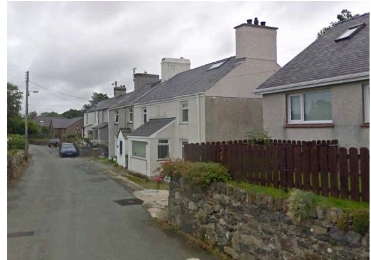
29 Modern porches, renders and uPVC windows have been installed to the detriment of the conservation area.
