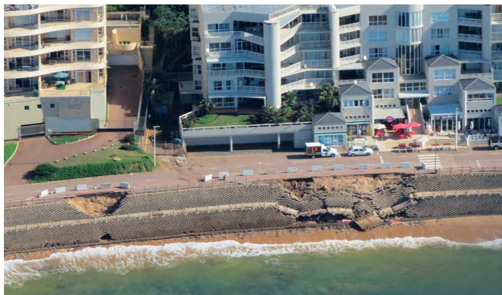
Coastal erosion at Umdloti Photo: ORI
