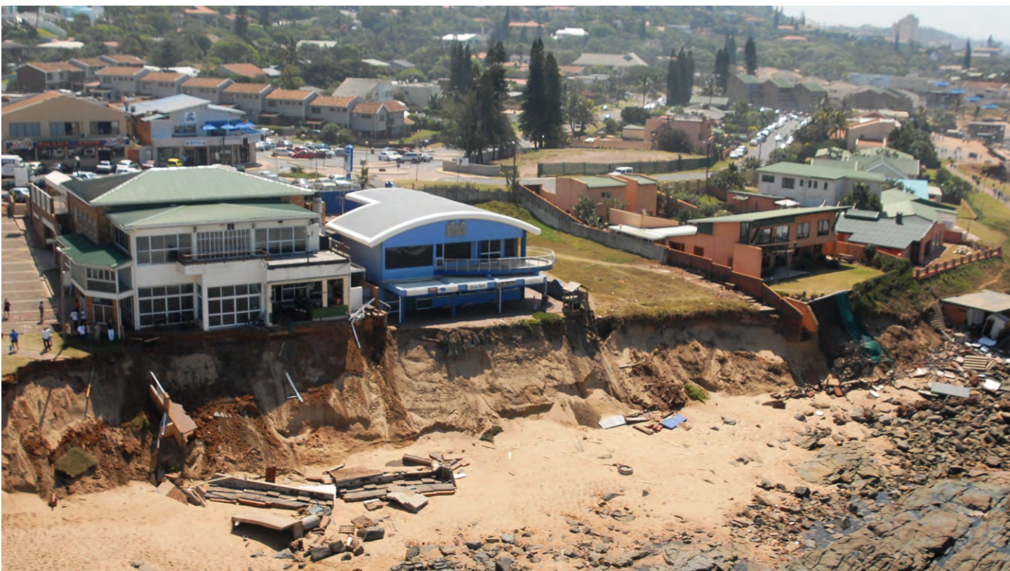
Erosion because of an extreme wave event Photo: Simon Bundy
