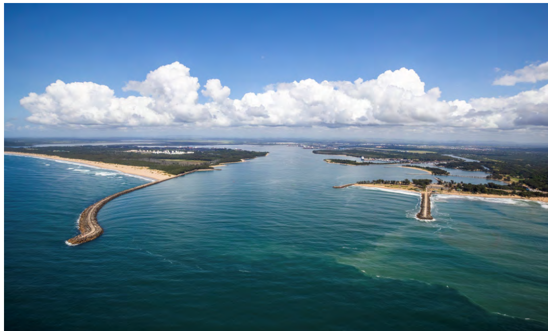
The Port of Richards Bay, KZN north coast. Photo: ORI
