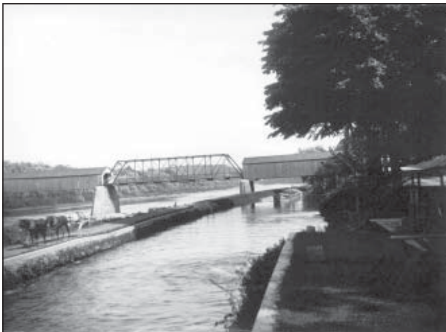
Vehicular bridge with steel span replacement section after flood of 1903. Note canal boat heading north. Photo by John A. Anderson, September 1910. Courtesy New Hope Historical Society.
