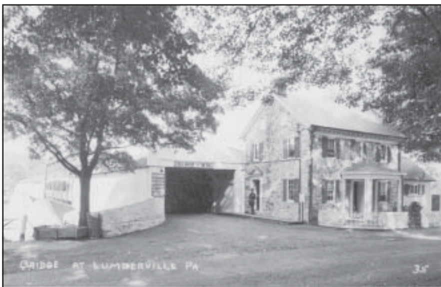
Bridge tender's house about 1935. 'Free Bridge – No Toll'. Steve Cohen collection.
