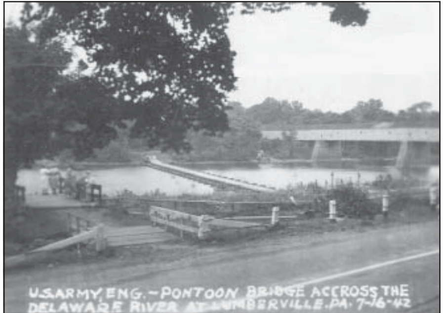
US Army Engineers – Pontoon Bridge Across the Delaware River at Lumberville, PA 7-16-42. Note canal lock to left; covered bridge to right. Tinsman Family collection.
