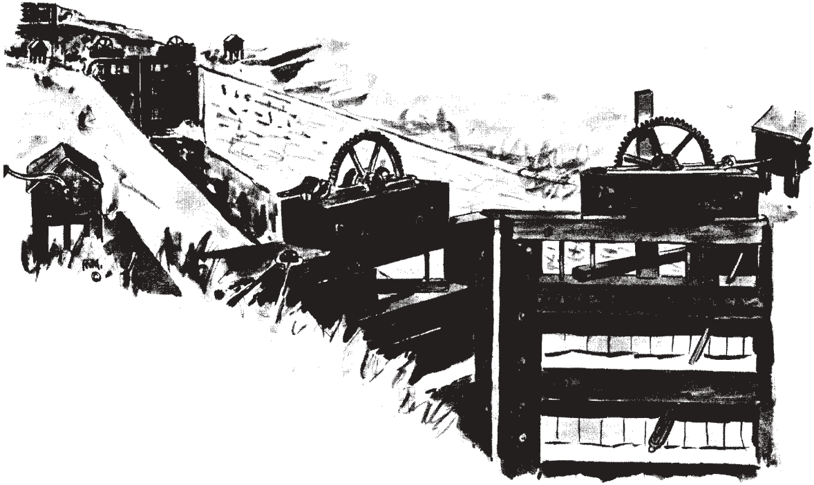
Canal Lock #12 at Lumberville. Unique 'dog house' at left controls the heavy wheels to raise and lower the gate's wickets. Sketch from The Delaware Canal by Robert J. McClellan.
