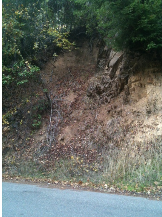
Figure 3: Evidence of potential LWM recruitment from landslides above Mill Creek Road.
