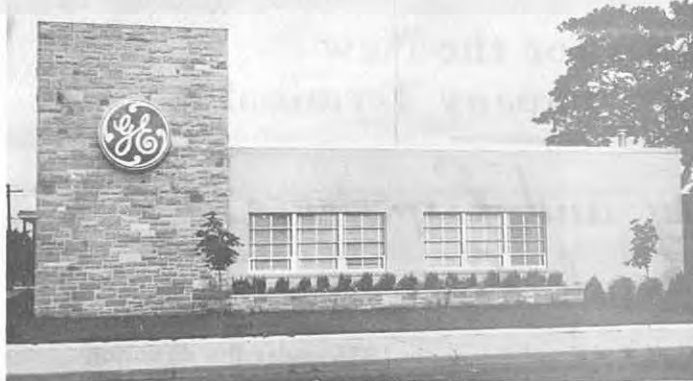
G. E. CO. SALES OFFICE & WAREHOUSE, PAWTUCKET, R.I., BY H.M. SOULE CO. ca.1959
