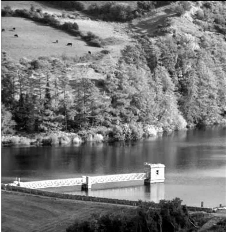
Upper Lake showing the valve house and dam.
