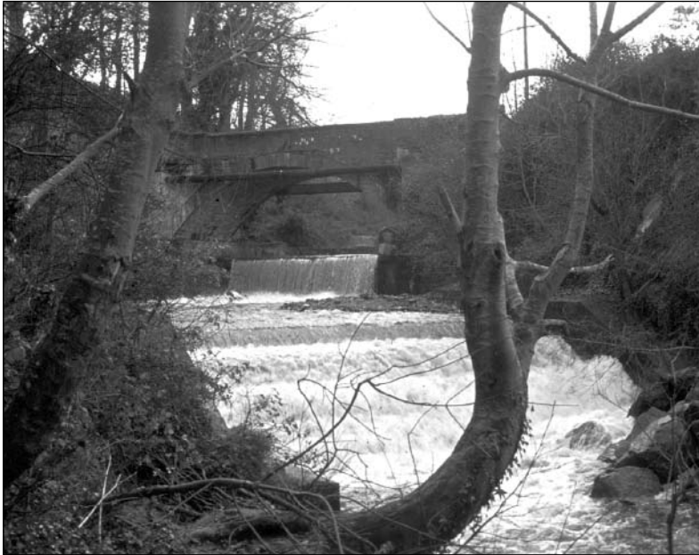
Fort Bridge, built after 1821 replaced a ford and a footbridge.
