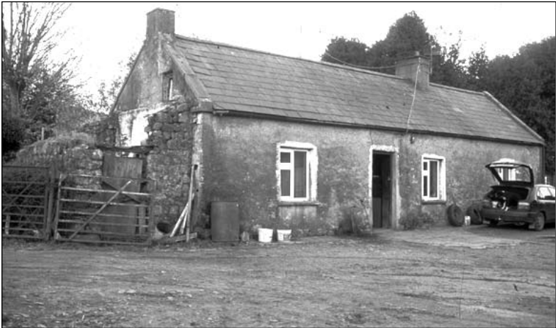
The house which was occupied by William Rafter in 1837. Courtesy of Tomás Maher.
