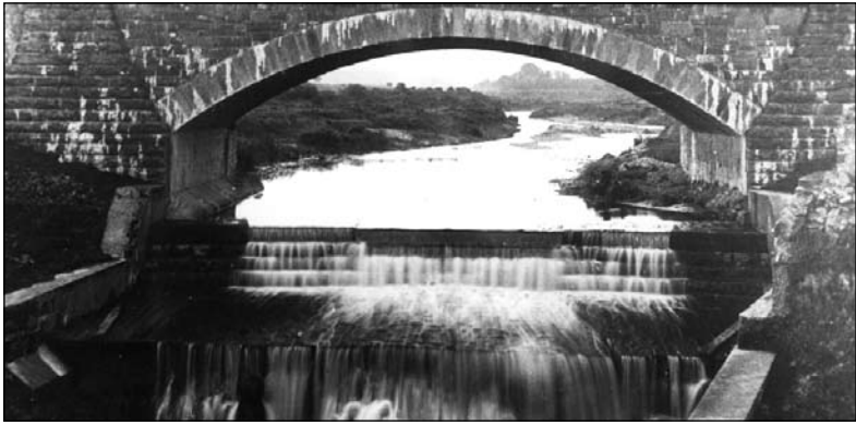
Old Bawn bridge
