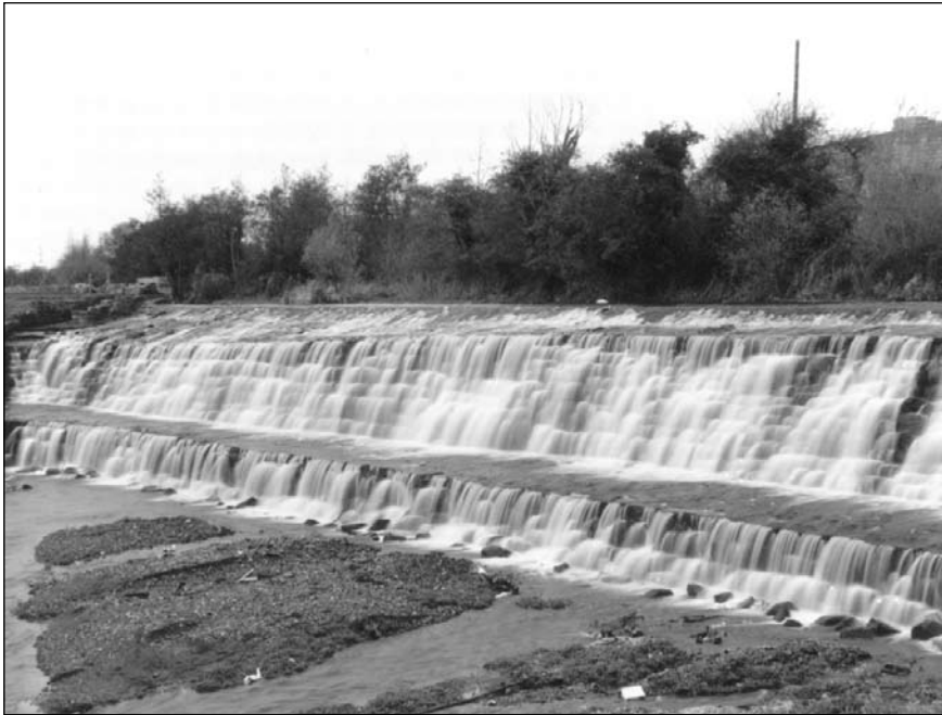
The City Weir at Firhouse
