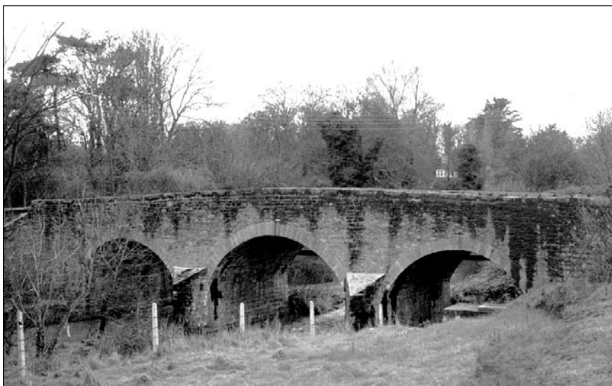
Templeogue Bridge was erected about 1800. Before this travellers who wished to cross the Dodder used a ford half a mile higher up the river — Patrick Healy
