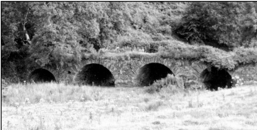
Downshire Bridge — Courtesy of Liam Roche
