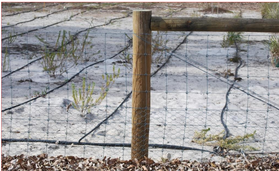
Figure 11: Ringlock fencing with treated pine posts
