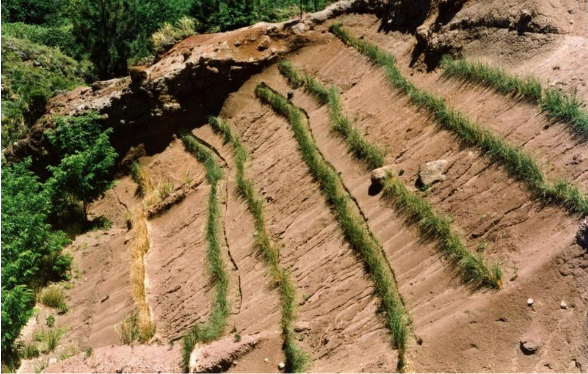
The successful slope plantings on a section of Chalk Hill, Aneityum, in 2001.
