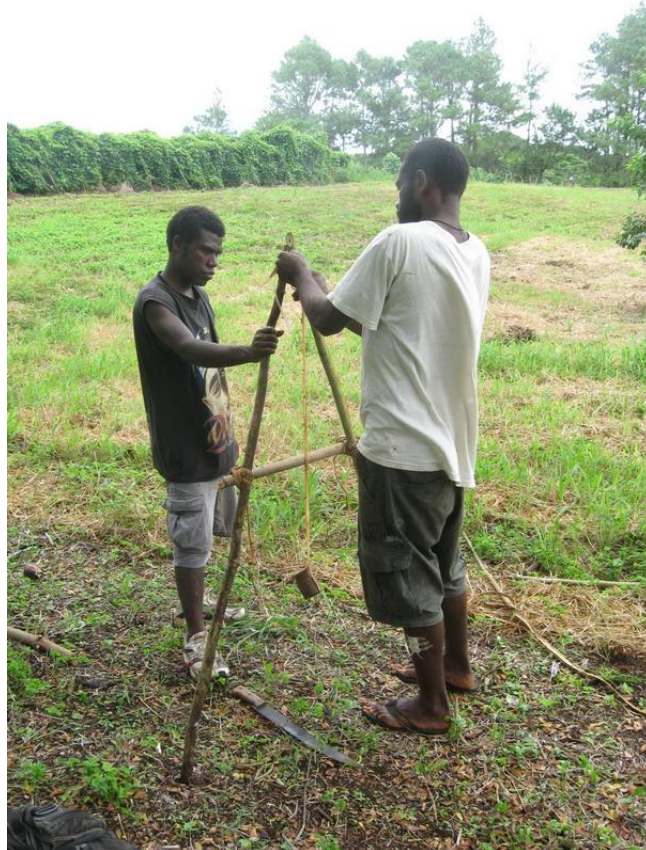
Building an A-frame level.
