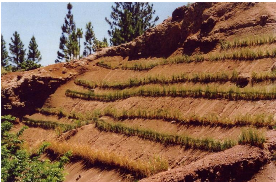
Initial contour rows of vetiver established on the gully walls in 2001.
