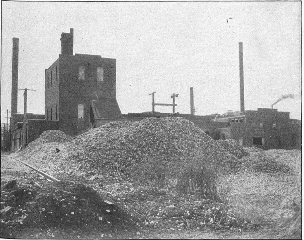
Crushing plant where waste shell and defective blanks are converted into chicken feed and other useful products. (See p. 80.)
