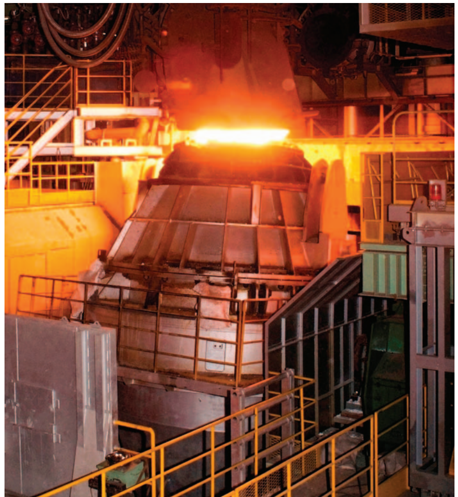
AVS equipment in operation producing Nippon Yakin's high performance alloys.
