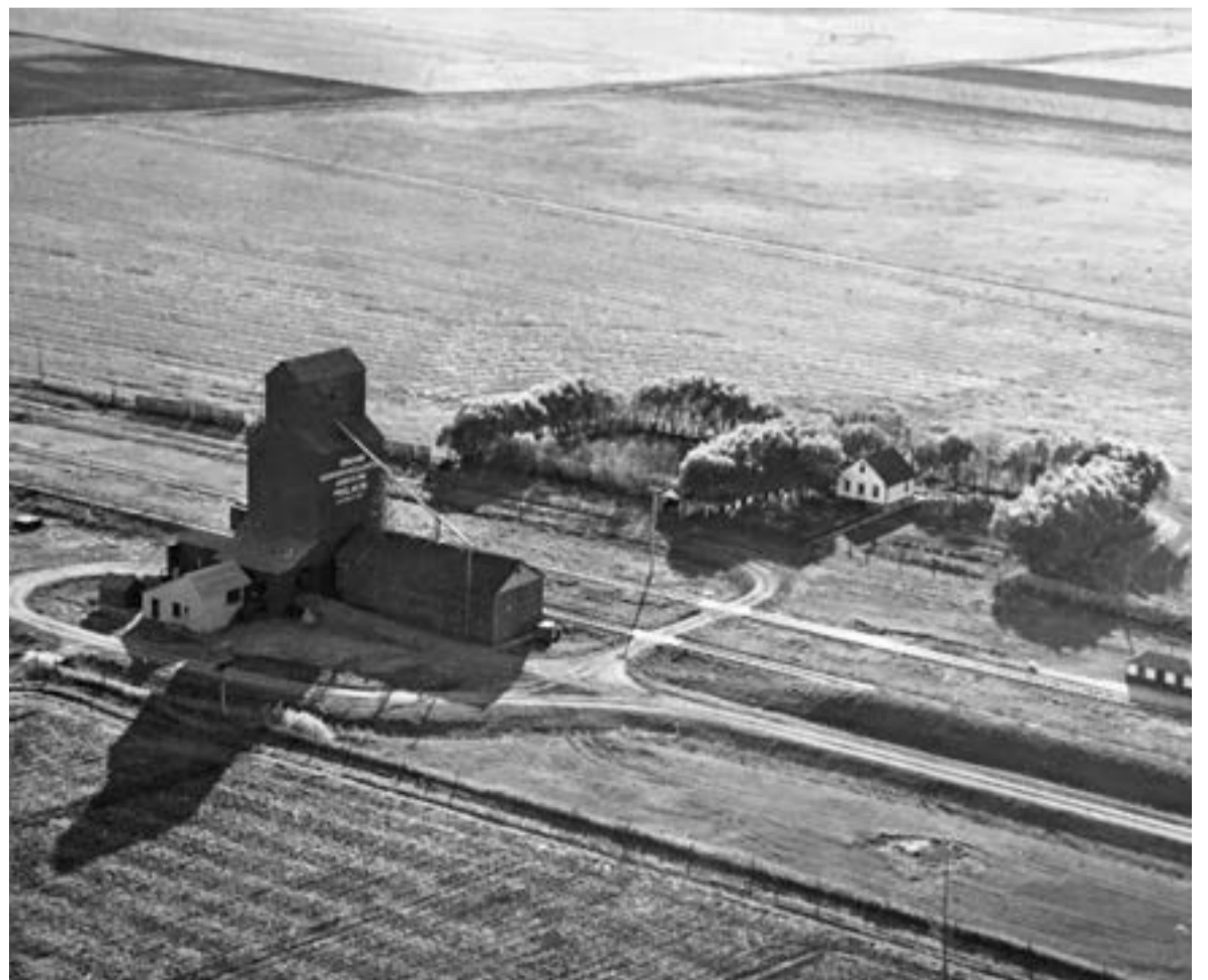
A 40,000-bushel wooden grain elevator at the railway siding of Graham, on the CPR Carman Subdivision in the Rural Municipality of Roland, was built in 1927 by Manitoba Pool Elevators. Closed in July 1971, the railway was abandoned in November 1975. No vestige of the railway tracks, elevator, agent’s residence, or access roads remain at the site in the middle of an agricultural field. This aerial view was provided by Doreen Smith whose husband Ralph was its agent from the mid-1940s to 1961.
