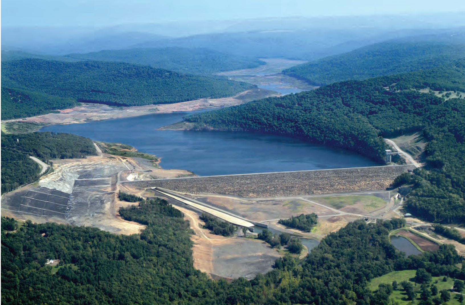
Aerial view of the recently completed $180 million Lake Fort Smith water supply project near Mountainburg. The raised and lengthened dam is in the center, the new water intake tower is at the far right, the spillways are at left center, and U.S. Highway 71 is at the far left, just out of picture.
