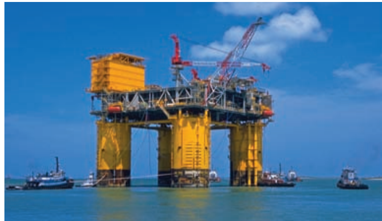
2004 | Above: The Magnolia extended tension leg platform (ETLP) is towed out into the Gulf of Mexico. The world's deepest ETLP at 4,698 feet, Magnolia's design capacity is an estimated daily production of 50,000 BBL of oil and 150 million cu. ft. of natural gas.
