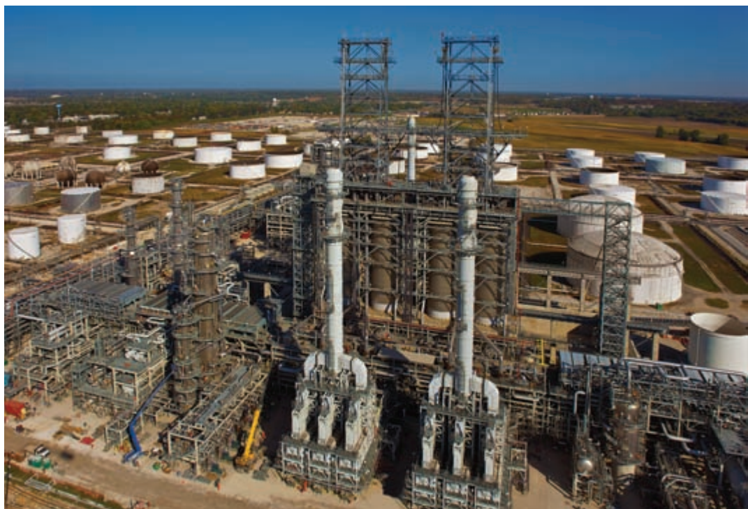
Below: The nearly completed CORE Project
