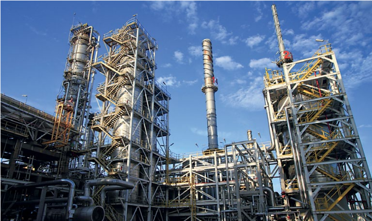
The Melaka Refinery saw a rise in crude oil throughput following the expansion of a hydrocracker and coker in 2010.
