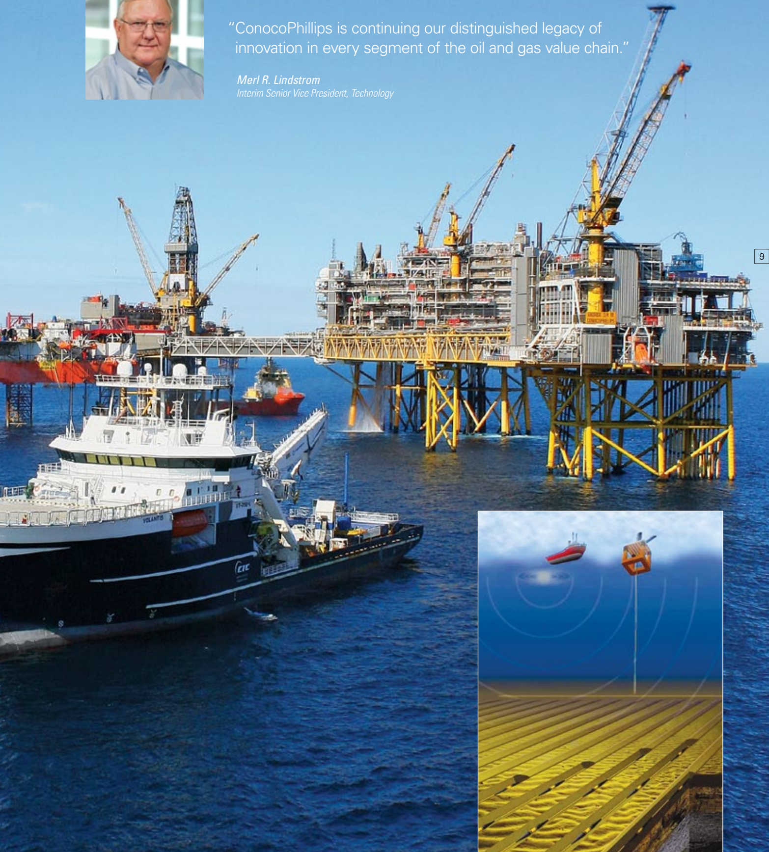
The installation vessel Volantis maneuvers through the Ekofisk Complex installing an ocean bed seismic array for a new Life of Field Seismic system designed to optimize management of oil reservoirs by creating a time-lapse measurement of reservoir fluid movements, known as 4-D seismic.
