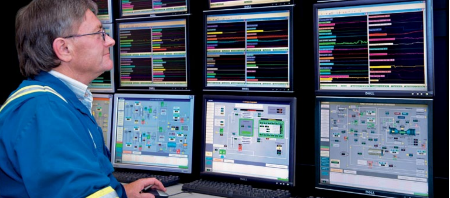
Advanced technology is being used to optimize returns from key legacy assets, such as in the Deep Basin in western Canada. Its gas and liquids are processed through multiple company-owned plants, including the Elmworth facility. ConocoPhillips is a leading producer in the basin.
