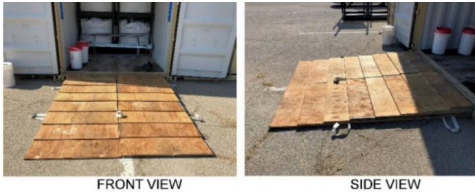
Figure 2.3. Expedient Ramp used to Unload Repair Material Containers.
