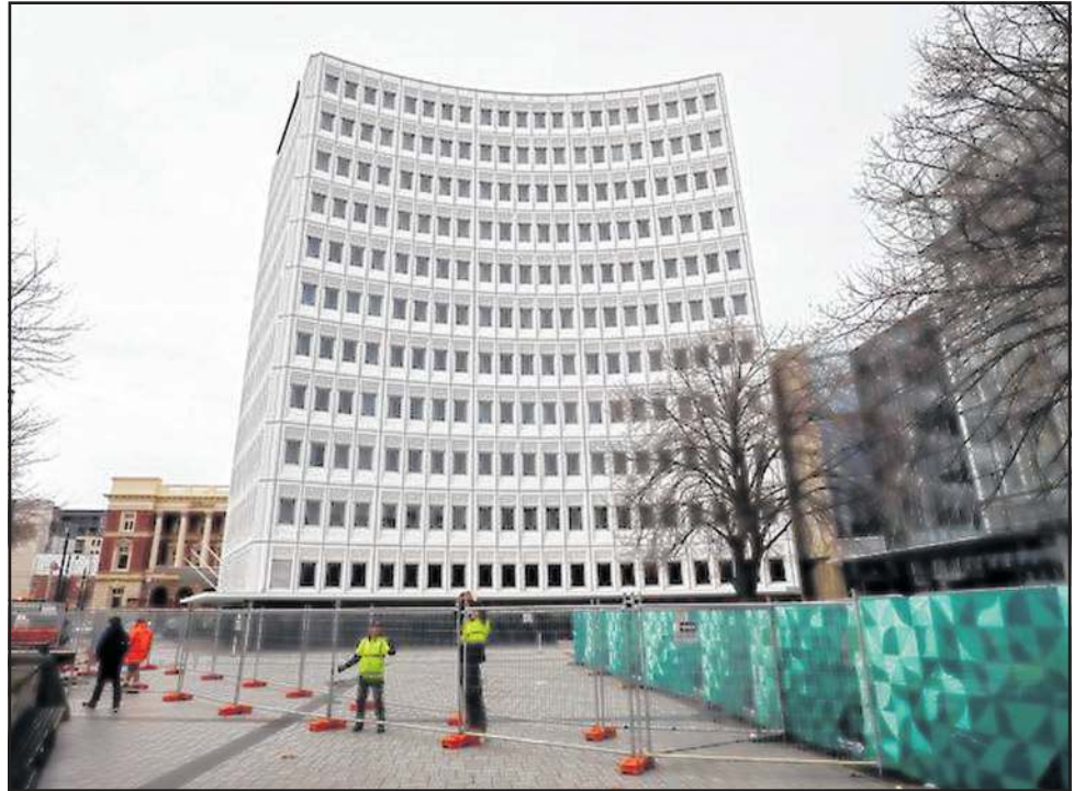
OVERLOADED: The Distinction Christchurch Hotel is one of the hotels being used as a managed isolation facility. RNZ picture
