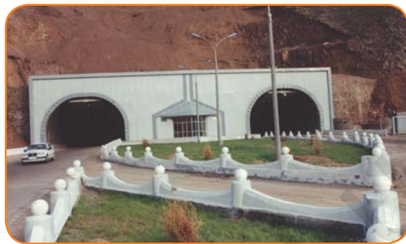
74-rasm. Qamchiq dovonidagi tunnel.
