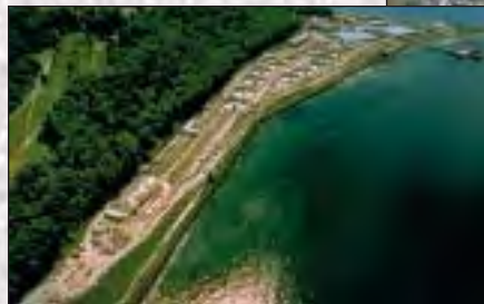
Water and Waste Water Treatment Plants
