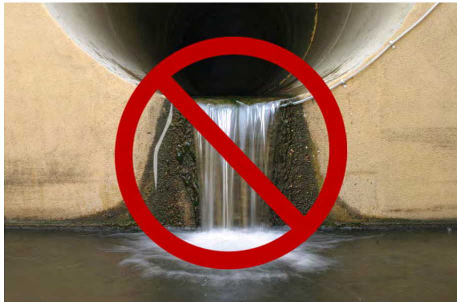
Figure B-1 Do not install LaserFlow with built-in sensor in a free-flowing outfall or in a drop manhole.
