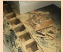
Severe Anobium punctatum damage.
