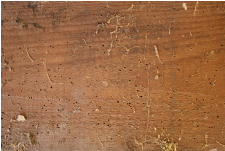
Severe Anobium punctatum damage.
