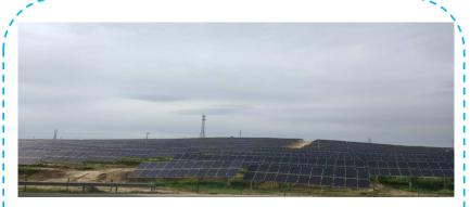
In late June 2016, we connected a 50 MW "Top Runner" project in Datong City, Shanxi Province to the grid. The project utilized Yingli's TwinMAX 60 Cell bifacial series module, a frameless dual glass module that integrates Yingli's cutting-edge PANDA (n-type monocrystalline solar cell) technology which leads to a module efficiency of up to 18.8%.
