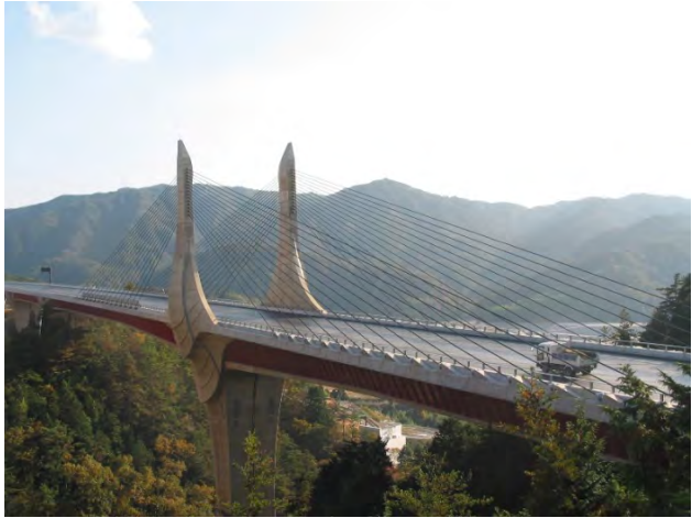
(a). Road (Ritto Bridge)
