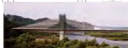
17 Yukizawa Bridge (雪沢大橋) 231+233 Japan 37.7 (2x2) 2000 (6.6-11.5)x51.8 Two cell concrete box girder
