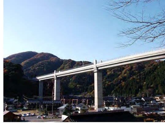
(b) New Amarube Bridge (Tower Height 16.5 Feet)
