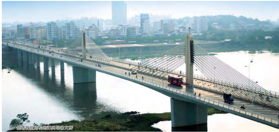
(a). Zhangzhou Zhanbei Bridge
