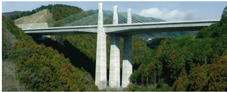
(a). Miyakoda River (Miyakodagawa) Bridge (1×3)
