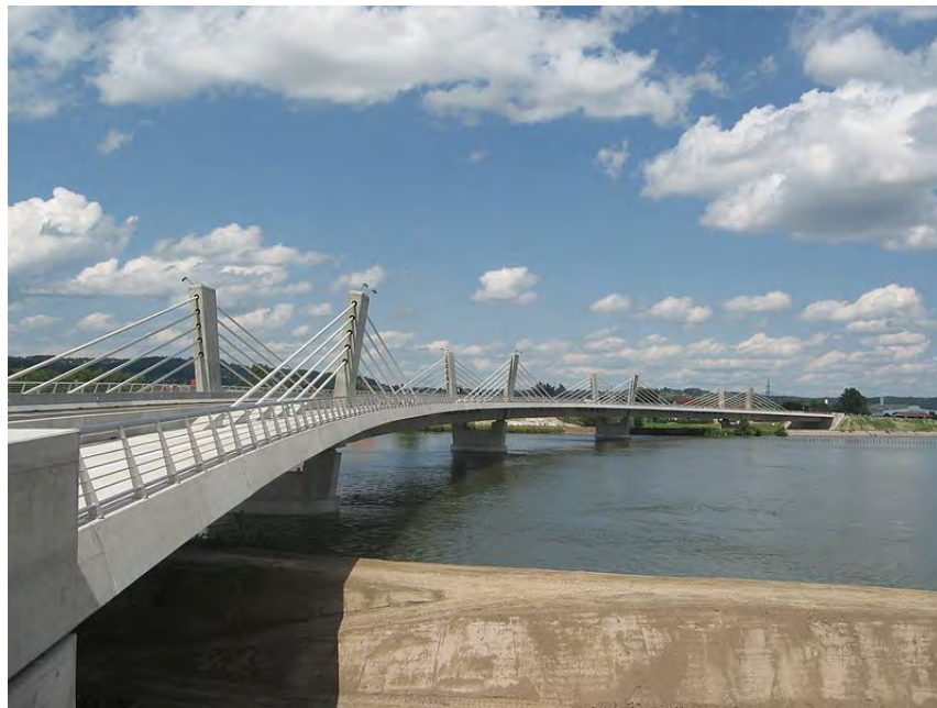
Figure 56. Example of Bridge with Proper Span for Curvature (Puh Bridge).
