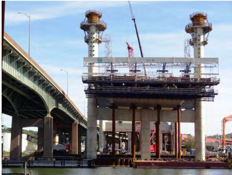
Figure 58. Example of Bridge with Construction Consideration (New Pearl Harbor Memorial Bridge).
