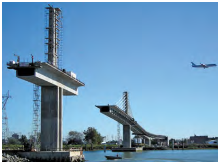
Figure 48. Example of Consideration of Aviation Restriction (North Arm Bridge).
