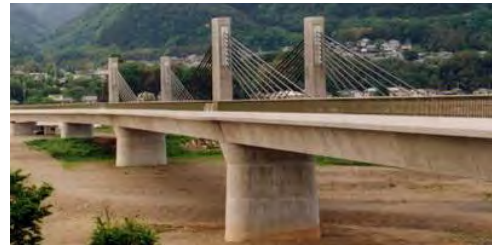
18 Hozu Bridge (保津橋) Japan 2001 249+328+249 32.8 (2x2) 9.2x53.5 Single cell concrete box girder
