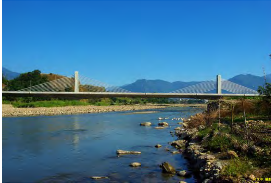
Figure 52. Examples of Bridges Selected due to Less Environmental Impact (Ailan Bridge).
