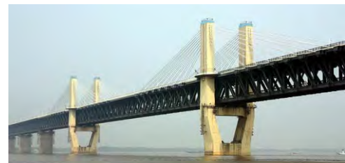
16 Wuhu Yangtze River Bridge (芜湖长江大桥) 591+1024+591 China 114.8 (2x2) 2002 (42) 44.3x76.8 Double-girderer steel truss with composite girder slab on top roadway, two rail lines on bottom level.
