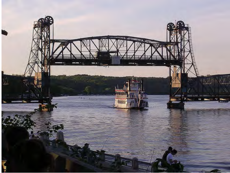
Figure 67. Stillwater Lift Bridge.
