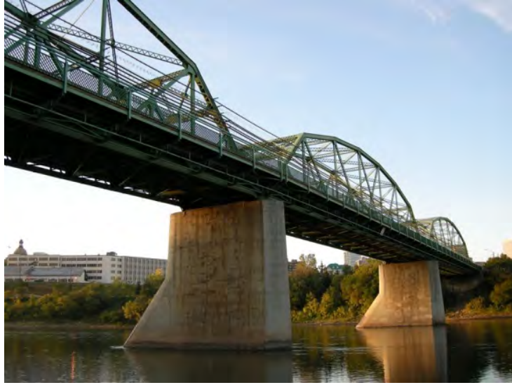
Figure 69. Existing Walterdale Bridge
