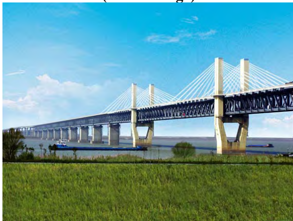
(c). Road and Railway Hybrid (Wuhu Yangtze River Bridge)
