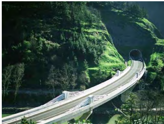
(b). Deba River Bridge
