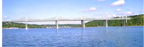
113 Saint Croix River Bridge United States 2014 290+6x480+290 60 (7x2) 16x110 Three cell concrete box girder (each direction)
