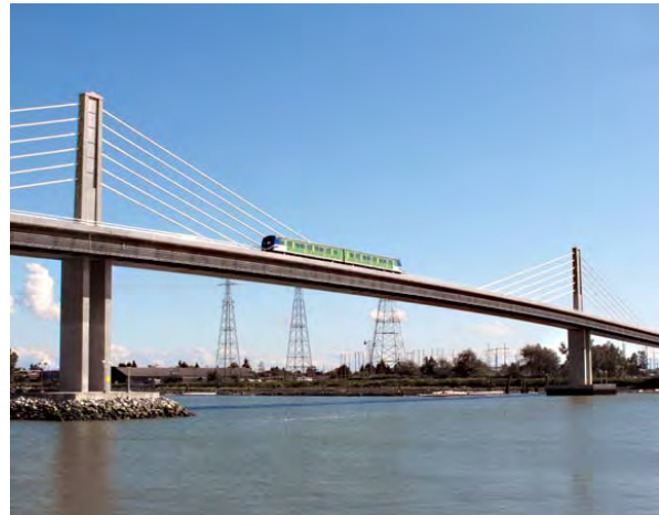
(b). Railway or Light Rail (North Arm Bridge)
