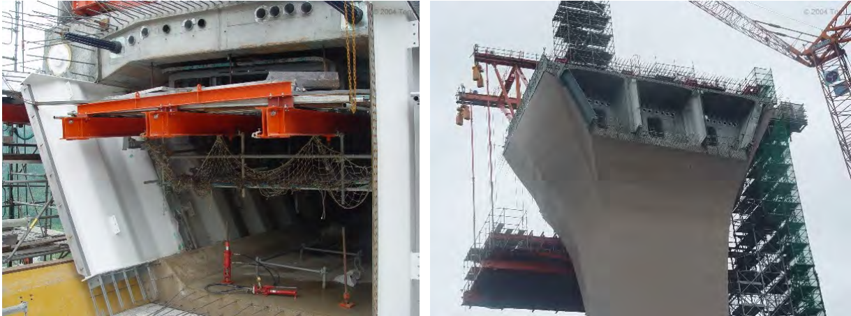
(a) Pylon and Pier Table
