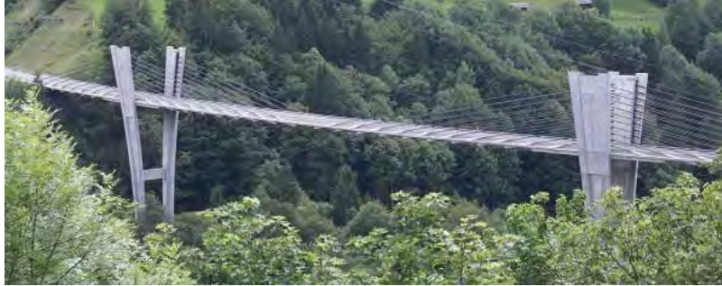
(a). Sunniberg Bridge (with Constant Girder Thickness of 3.6 Feet)
