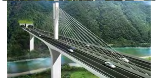
116 Naerincheon Bridge Korea 2015 394+509 -(1x1) -x100.1 Concrete box girder
