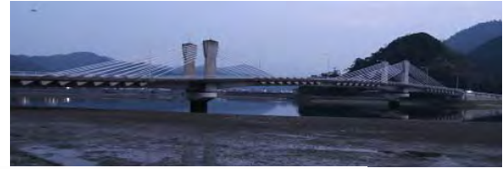
13 Sajiki Bridge (佐敦大桥) 201+344+191 Japan 38.5 (2x2) 2000 (6.9-10.5)x36.1 Concrete box girder
