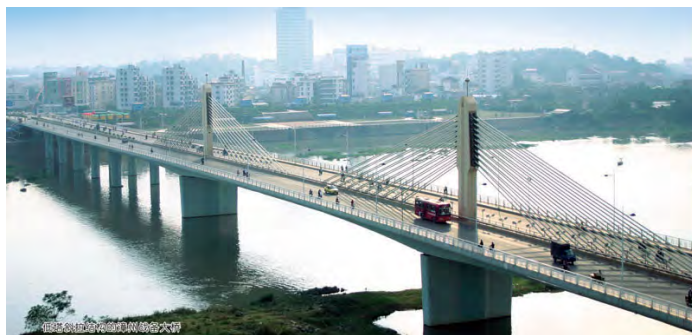
(c). Zhangzhou Zhanbei Bridge (2×1)
