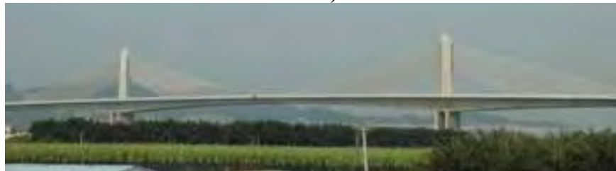
(d). Panyu Shawan Bridge (with Variable Girder Thickness of 13.1 Feet at Midspans and 27.9 Feet at Piers)
