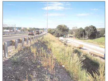
The 2:1 MSE slope at Marston Street was steepened to 1:1.
