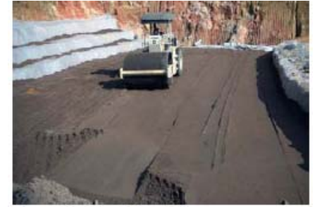
Compacting the reinforced fill
