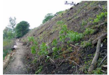
Clearing of vegetation from the existing embankment slope
