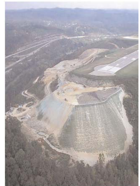
Aerial photo of slope during construction, approximately 80% complete.
