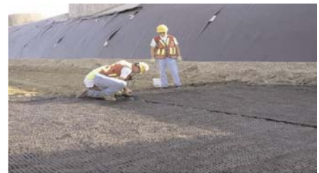
Installing stakes to keep geogrid positioned.
