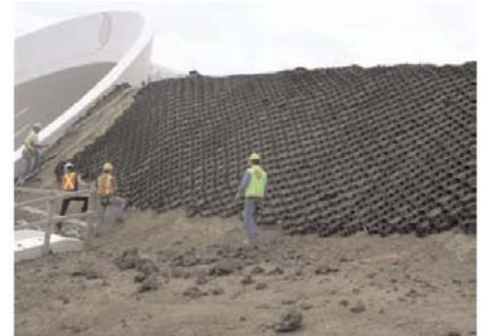
Above: 10cm (4in) Geocell material being installed.
