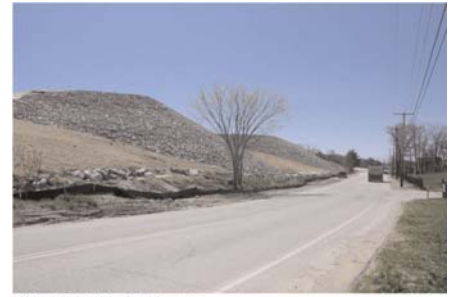
ABOVE: The finished Miragrid® reinforced slopes.
