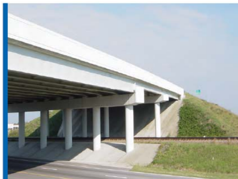
The completed Clemson Road bridge abutment.
