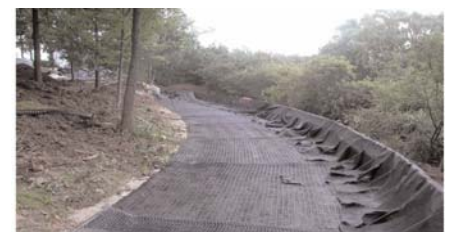
Miragrid® 150N separates the topsoil and granular reinforced zone.
