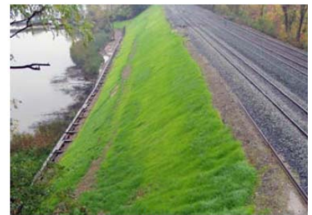
Completed reinforced fill slope with vegetated surface
