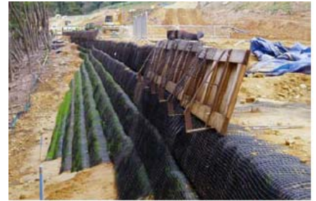
Use of timber shutter system to align the face for the steep reinforced slope sections
