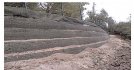
Miramesh® GR is selected as the face wrap to protect the vegetation from erosion.
