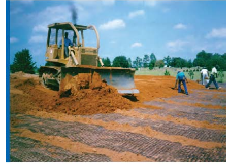
Fill is placed atop StrataGRID in the Reinforced Structured Slope.
