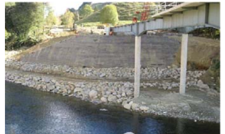
Completed Green Terramesh abutment structure Date: April 2009
