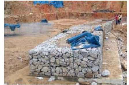
Installing the gabion toe of the reinforced slope
