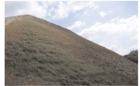
Completed 242 foot slope with good vegetation cover.
