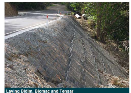
Laying Bidim, Biomac and Tensar
