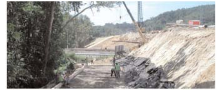
Preparing the drainage fabric behind the slope.
