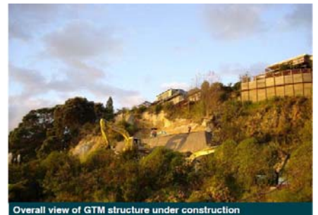
Overall view of GTM structure under construction
