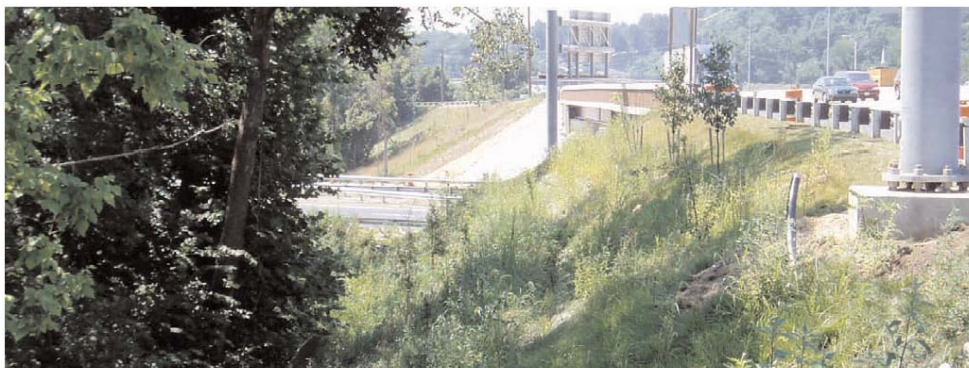
Completed slope with vegetation.
