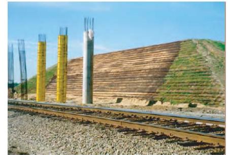
Construction of the StrataSLOPE for the Clemson Road project.
