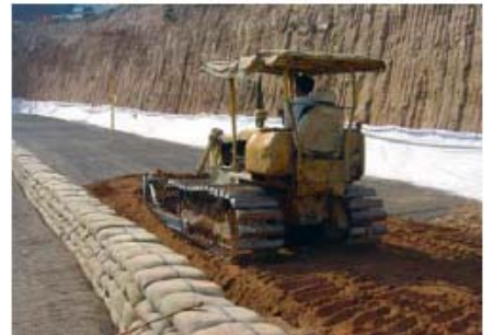
Spreading locally obtained reinforced fill over Miragrid® GX geogrid reinforcement
