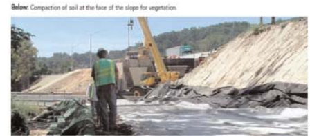
Below: Compaction of soil at the face of the slope for vegetation.
