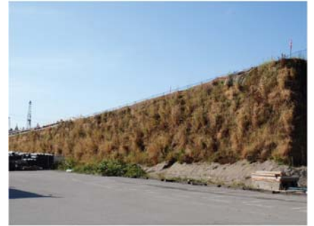
Nearly two dozen Sierra Slopes were installed as part of the Port Mann Bridge Project. The bridge will double existing lanes from five to ten and will sustain Vancouver's traffic growth over the next two decades.
