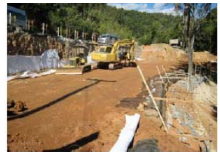
Placing reinforced fill in the reinforced slope
