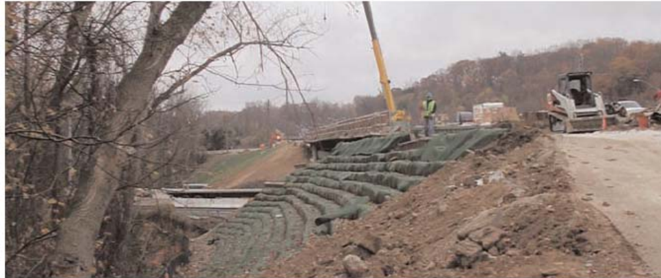
Slope nearing the finished grade.
