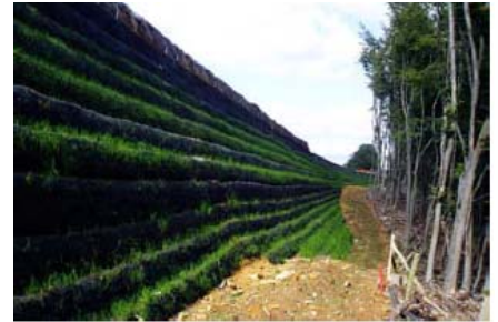
One of the steep reinforced slopes nearing completion
