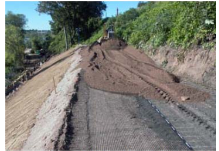
Placing reinforced fill over Miragrid® XT geogrid reinforcement
