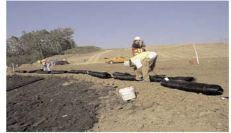
Pre-cut lengths of 21m (69ft) Miragrid® 10XT geogrid ready to be rolled out.
