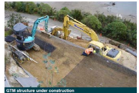
GTM structure under construction
