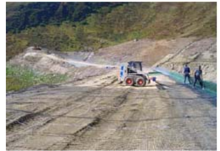
Miragrid® GX geogrid reinforcement being placed in the reinforced slope
