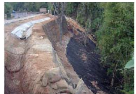
Reinforced slope nearing completion
