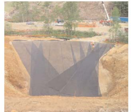
First layer of Miragrid® 24XT placed at base elevation.
