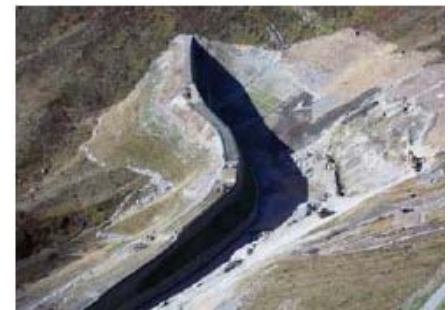
Avalanche protection barrier almost completed
