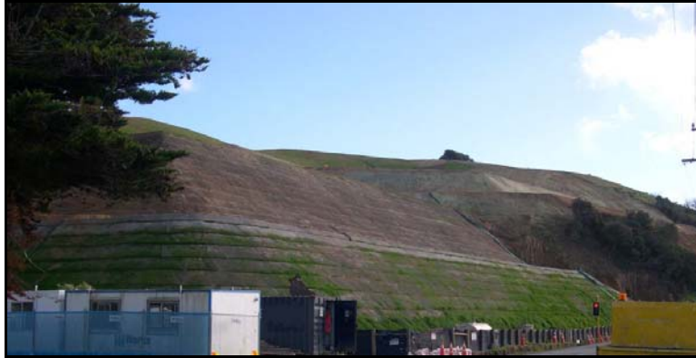
Figure 26. Vegetative Cover of Geosynthetic Reinforced Steep Slope.
