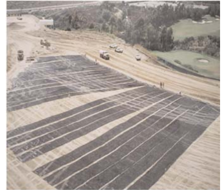
Over 400,000 yds 2 of Miragrid® geogrids were used to reinforce this development.
