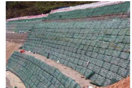
Reinforced slope partially completed
