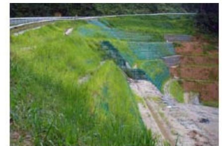
Completed reinforced slope with vegetation being established
