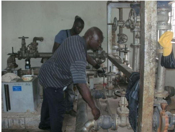
Figure 11 - Rokupr Water Works
