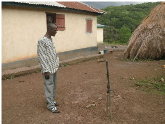
Figure 22 - Public water tap in Fintonia
