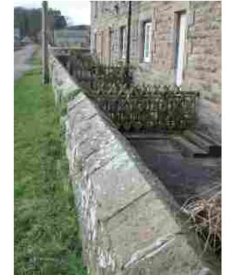
Figure 55: Saddle (pointed) coping stones, North Charlton
