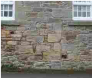
Sandstone rubble wall
