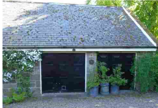
Figure 36: Garage at property in Eglington
