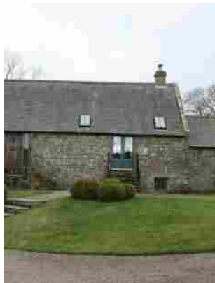
Small chimney and skylights
