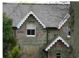
Decorative painted soffits
