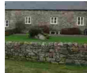
Sandstone boundary wall
