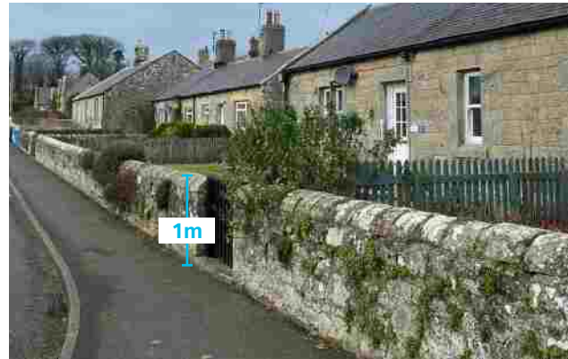
Figure 56: Consistent boundary wall frames the street, South Charlton
