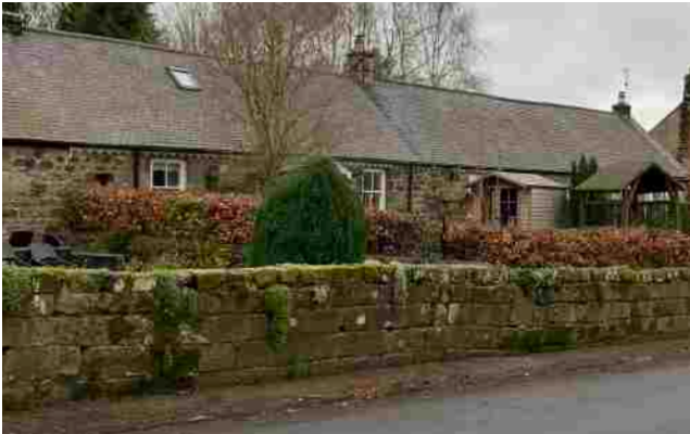
Figure 44: Short terraced row of bungalows with gable roof and stone chimneys, Eglingham
