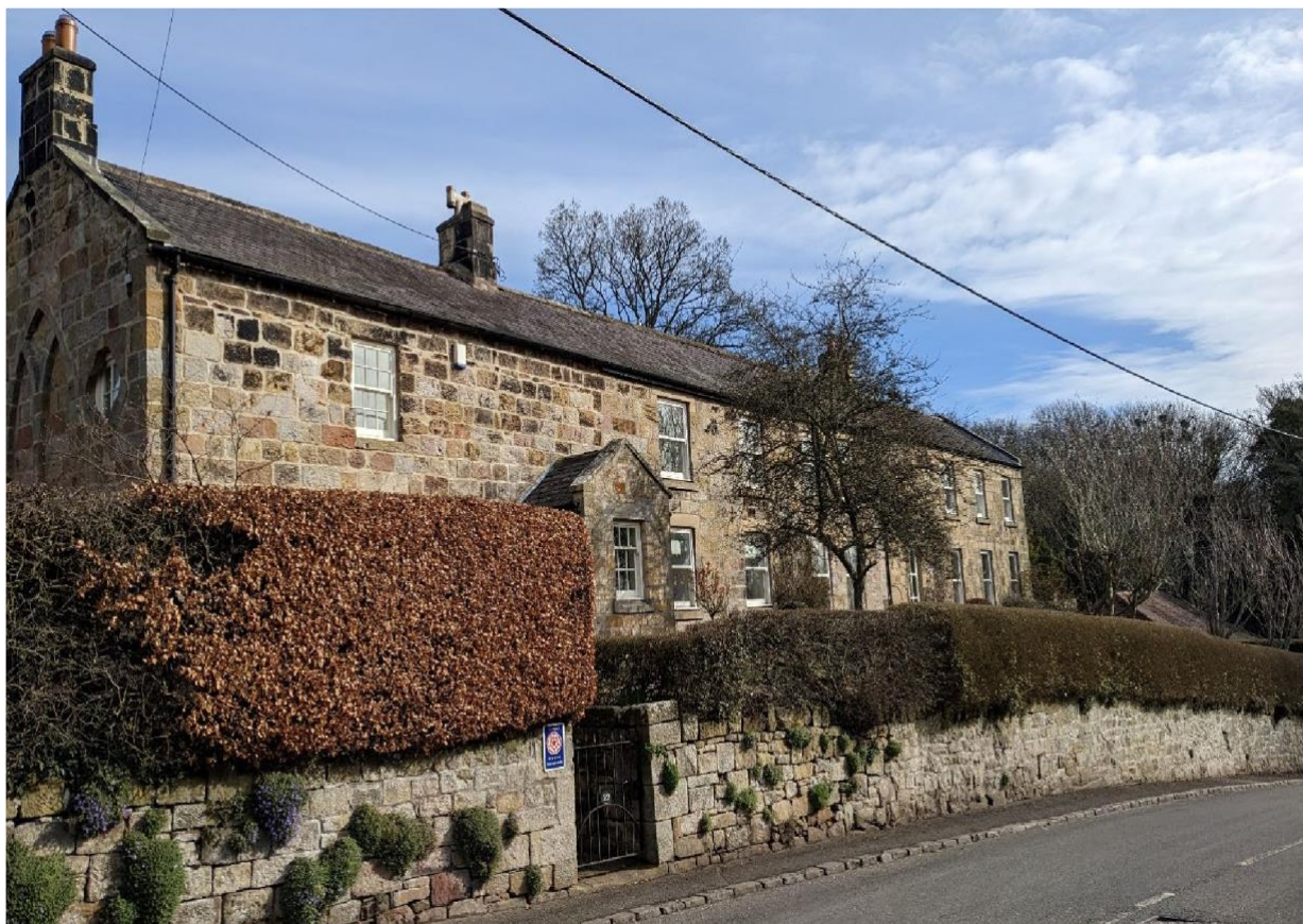
Figure 3: Typical building styles in Eglingham showing square coping to boundary walls
