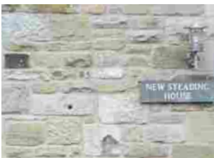
Mortar tone matches sandstone
