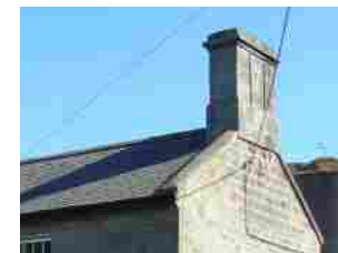
Rectangular chimney stack
