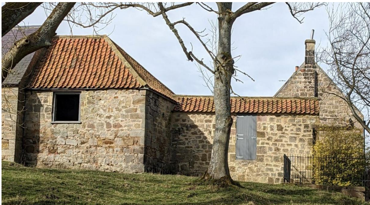
Figure 5: Village Farm, Eglingham - From Bridge
