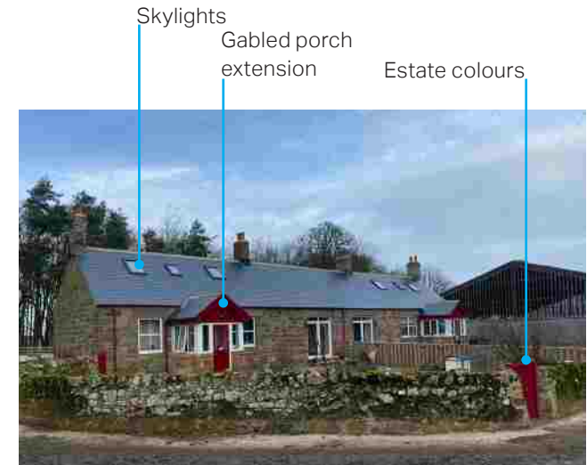
Figure 51: Renovated workers cottages, West Ditchburn
